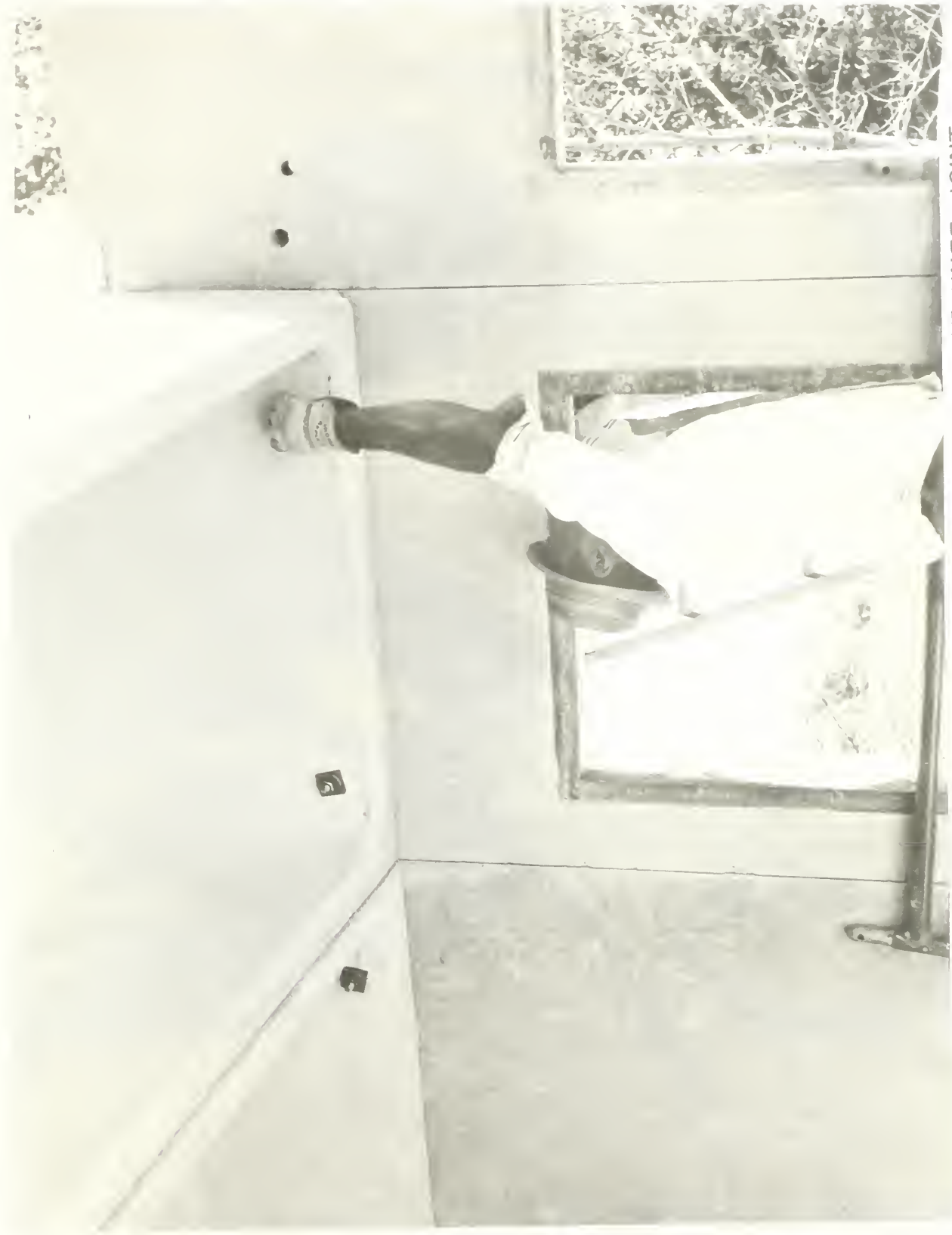
FIG. 5. BOLTING ROOF TO SIDE WALL PANELS AT KNEE JOINT
