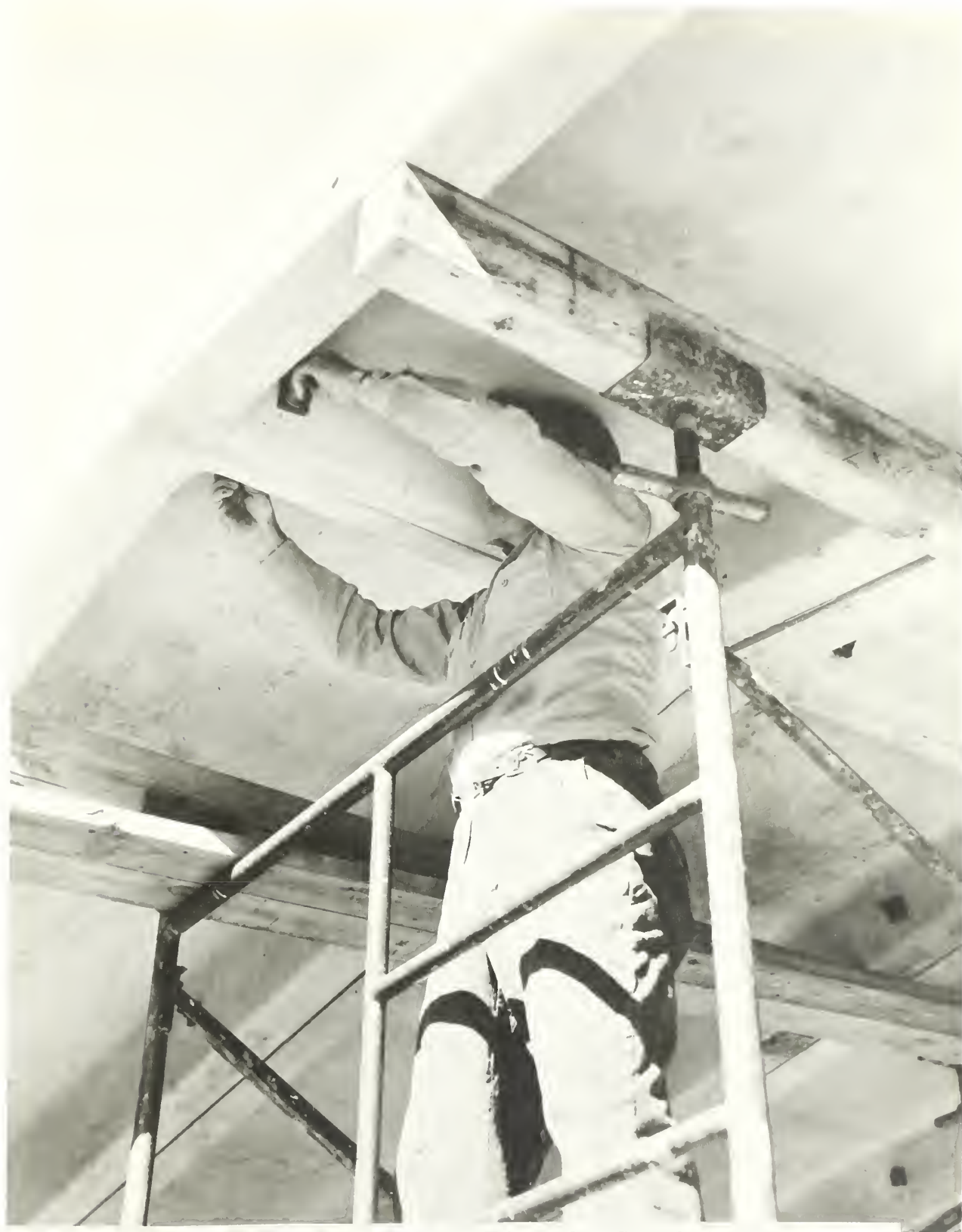
FIG. 4. BOLTING ROOF PANELS TOGETHER AT RIDGE JOINT
