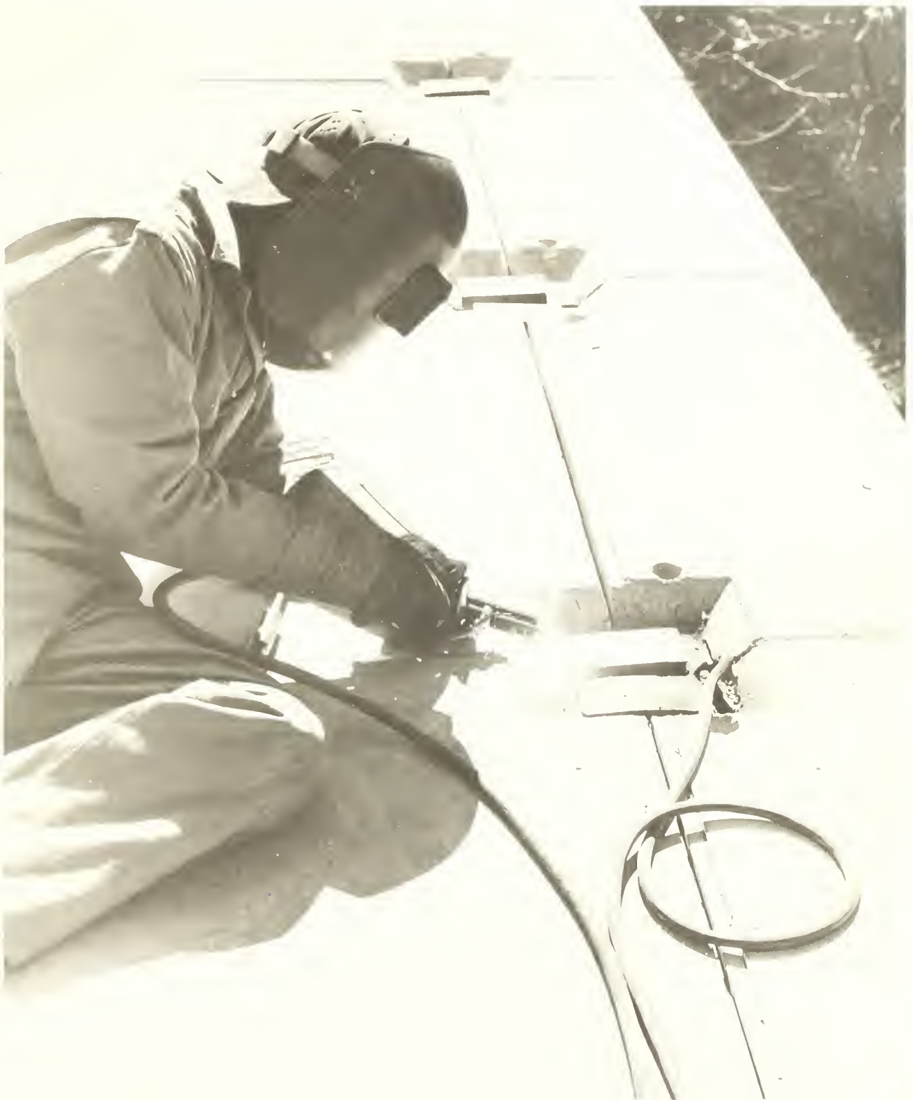
FIG. 6. WELDING ROOF TO SIDE WALL PANELS AT KNEE JOINT
