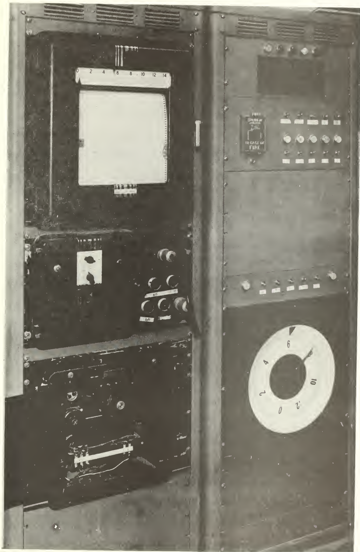
Fig. 8 Furnace Program Control Unit
