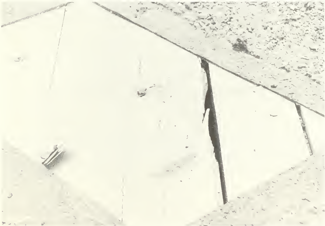
FIGURE 3. AFTER REMOVAL OF SPECIMEN.
