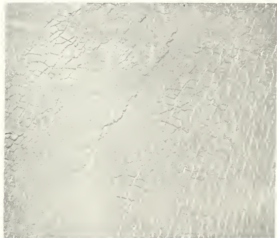
FIGURE 9. CRACKING IN FELT.
