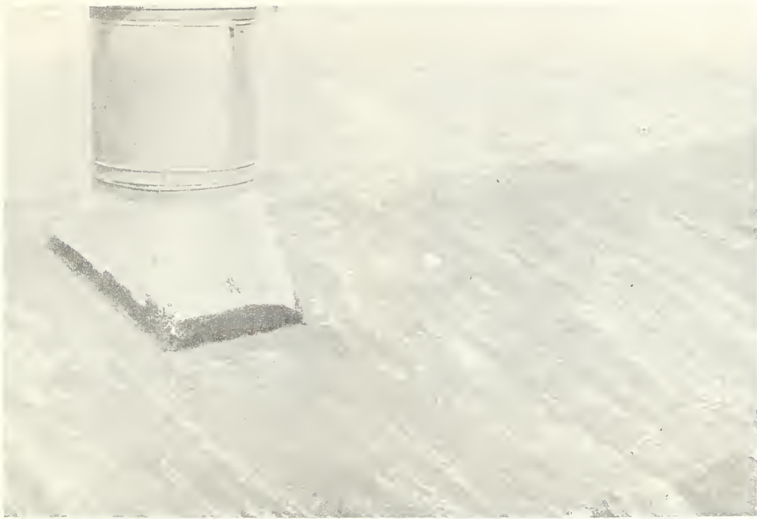
FIGURE 4. BUILT-UP ROOF APPLIED TO CORRUGATED METAL DECK.
