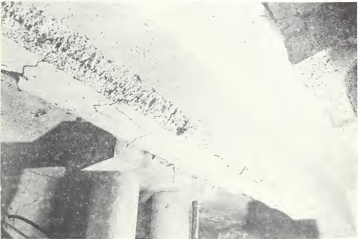
Figure 4. Fairly heavy and extensive sloughing from beam despite presence of wire fabric.
