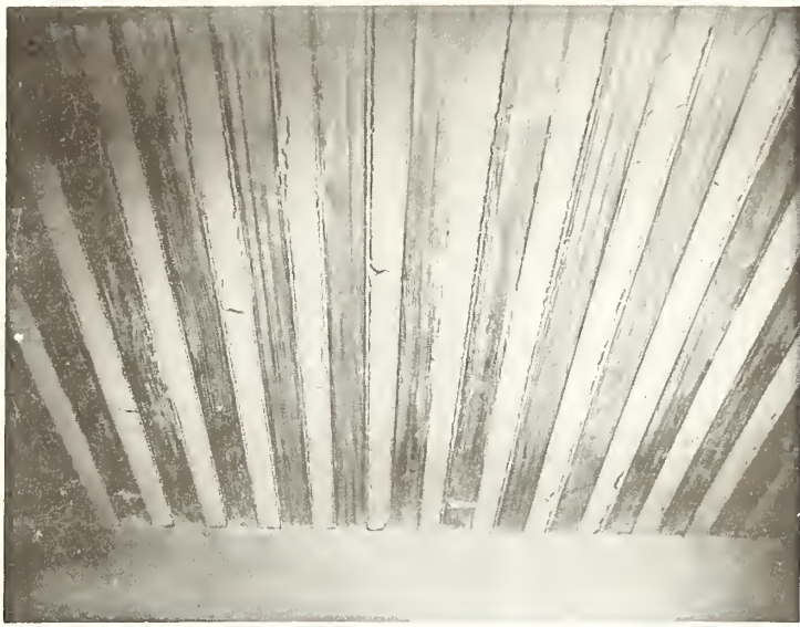
Fig. 2. Shrinkage cracks one week after initial application of acoustical plastic to fill between-cell spaces.
