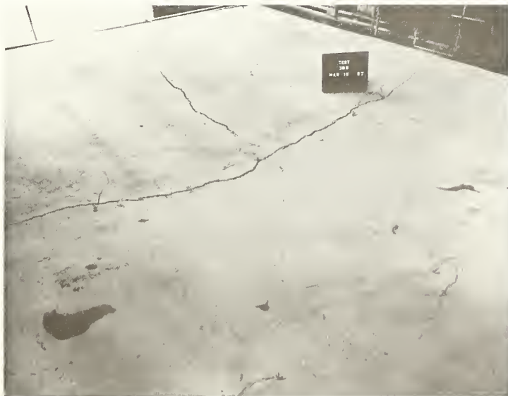
Fig. 4. Condition of unexposed surface after cooling and removal of loading apparatus.
