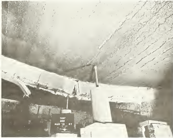
Fig. 3. Condition of exposed surface after fire exposure and cooling.
