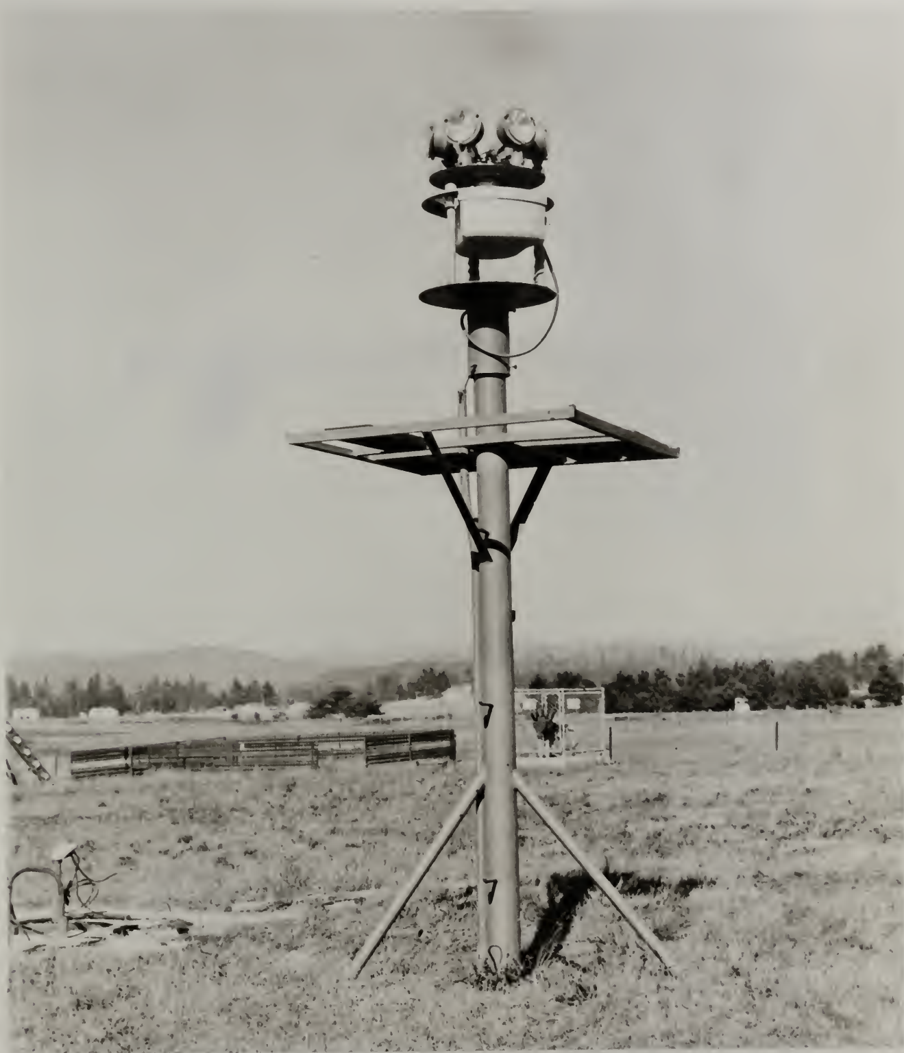
APPROACH BEACON INSTALLATION
