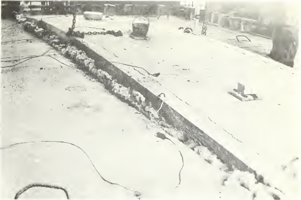
Fig. 5. Arched condition of panel, test 364, tested without applied load.
