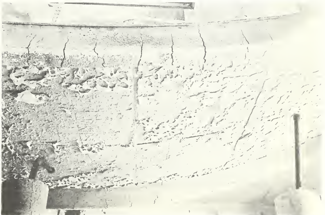
Fig. 6. Exposed surface of specimen having had glass fiber underface, showing remains of same and cracks in concrete.
