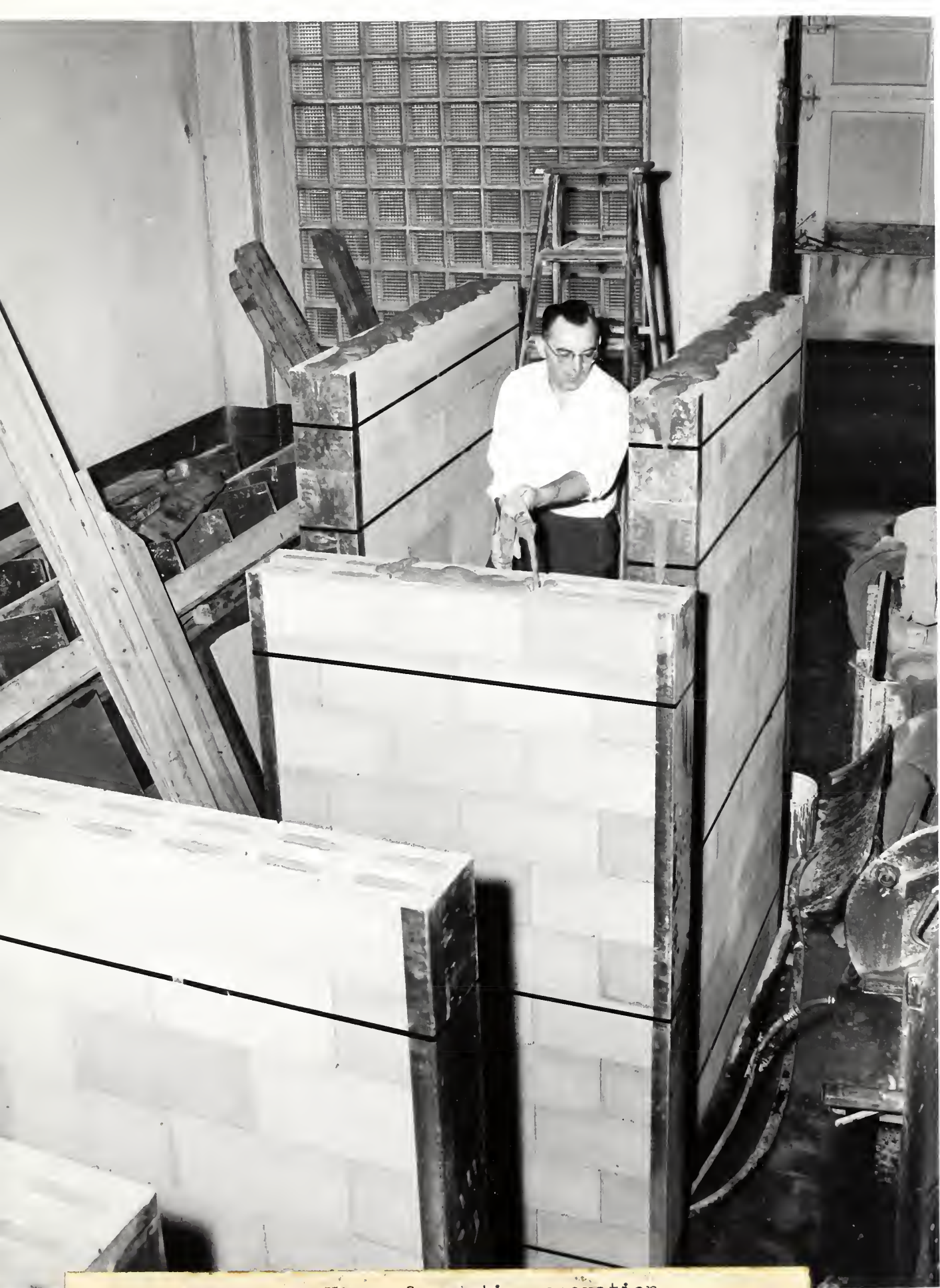
Fig. 3 - View of grouting operation.
