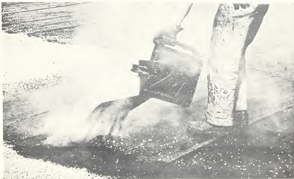
Figure 13. Laying felts mechanically and brooming in after felt is rolled into hot bitumen.
