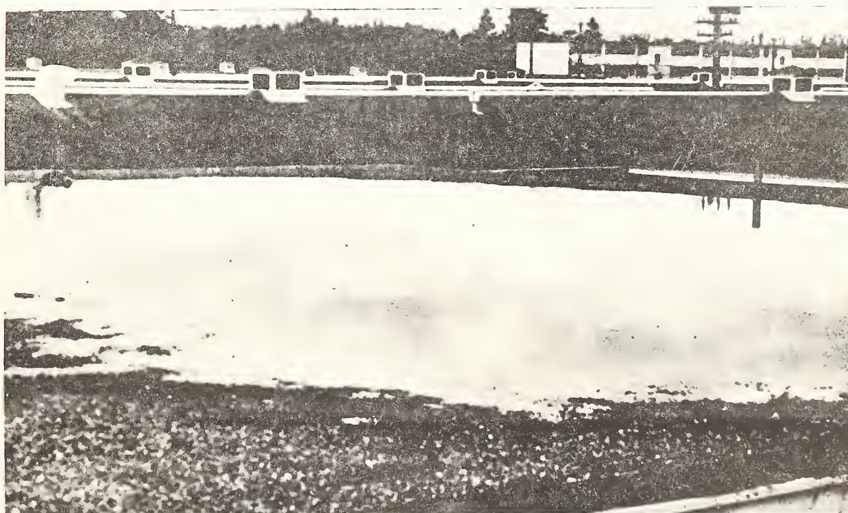
Figure 47. Standing water resulting from structural defect.
