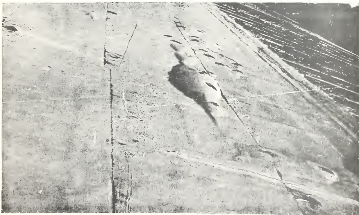
Figure 26. Large blister on smooth-surfaced roof.
