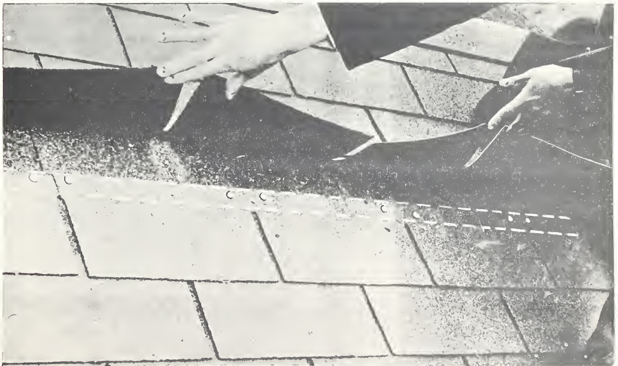
Figure 32. Proper nailing of asphalt shingles.
