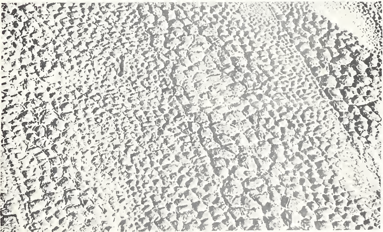
Figure 22. Alligatoring and cracking of a cold coating over alligatorated asphalt surface after one year exposure.
