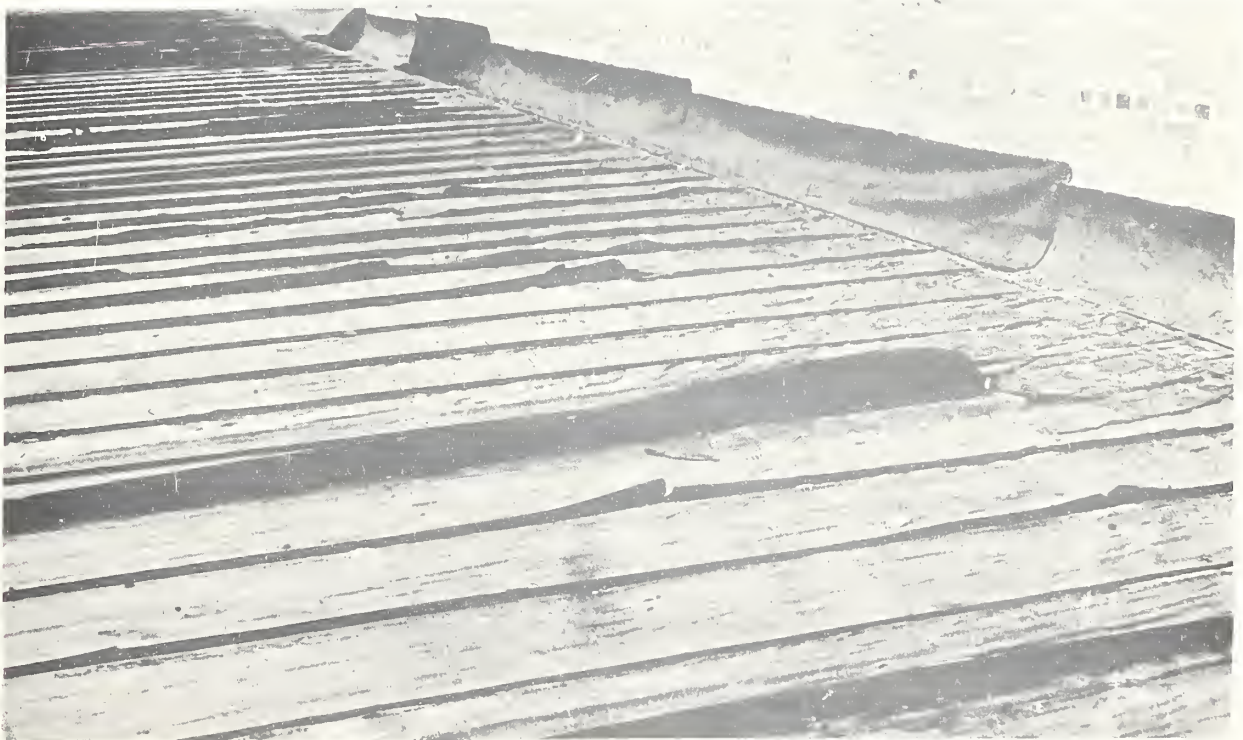
Figure 11. Leaks caused by entrance of water at defective flashings are sometimes attributed to failure of roof membrane.
