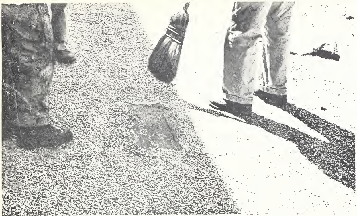
Figure 15. Insufficient bitumen to embed mineral surfacing.
