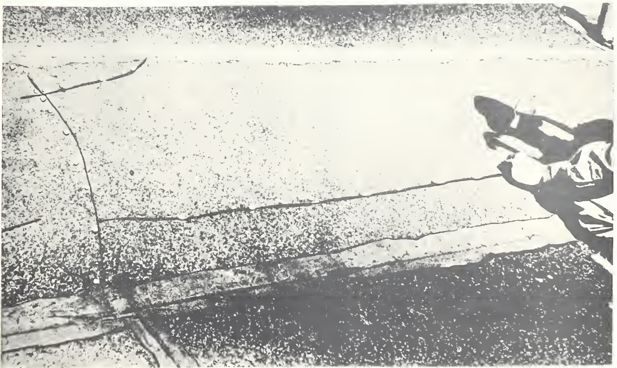
Figure 36. Buckles and wrinkles in existing roofing must be cut and edges nailed down to obtain a flat surface for application of a new roof.
