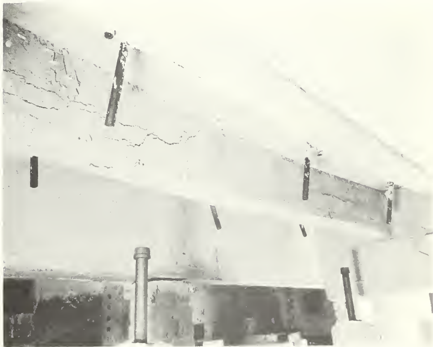
FIG. 7 A:1/2:0 BEAM AFTER FIRE TEST 331 AND RELOADING TEST
