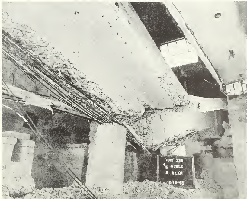
FIG. 9, D 4 / 5 -0 BEAM AFTER FIRE TEST 332, SHOWING BREAKS IN SLAB, BEAM, AND CABLE, THE LATTER GROUPED IN TWO LOCATIONS.
