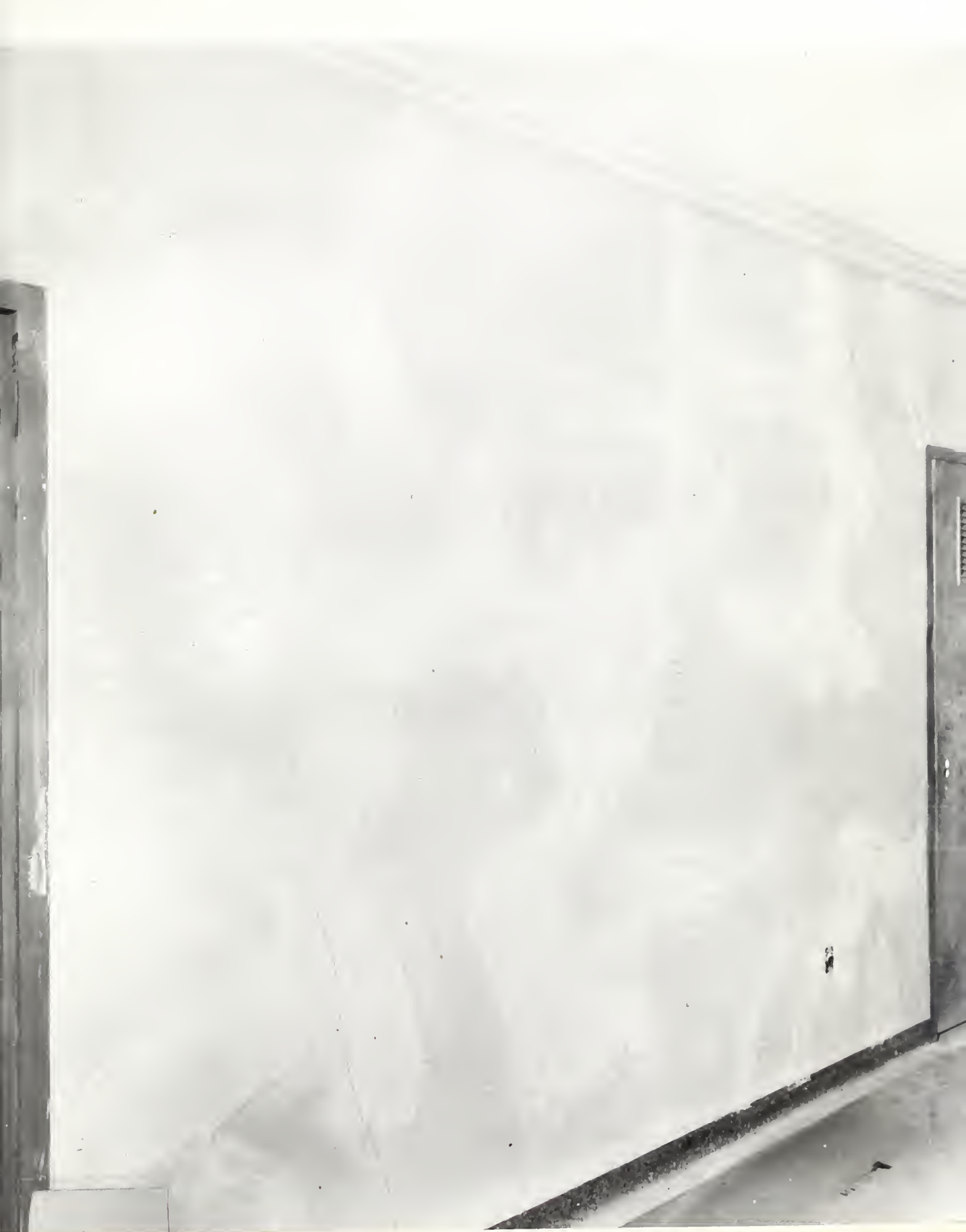
FIGURE 4. PROJECT 501-228. CORRIDOR E-501; 99% OF CRACKS THROUGH TO LATH. THIS WALL REQUIRED 73 LIN. FT. OF REPAIR ON 9-BY 10-FT. AREA SHOWN.
