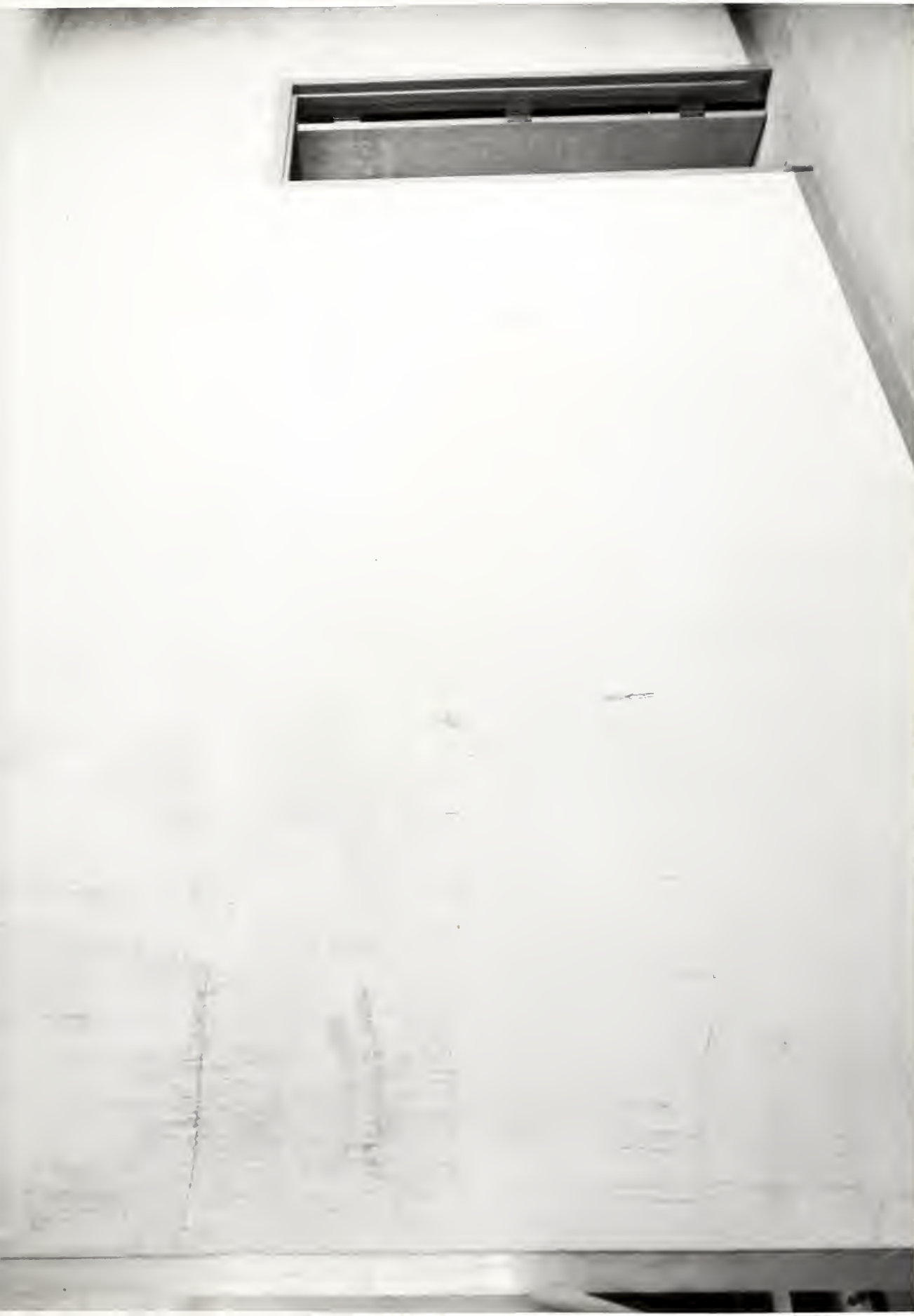
FIGURE 8. PROJECT 501-228. S-100, ( SOUTH CORRIDOR ) NEAR LAUNDRY ENTRANCE SHOWING CONDITION OF PLASTER ON OCTOBER 22, 1952.
