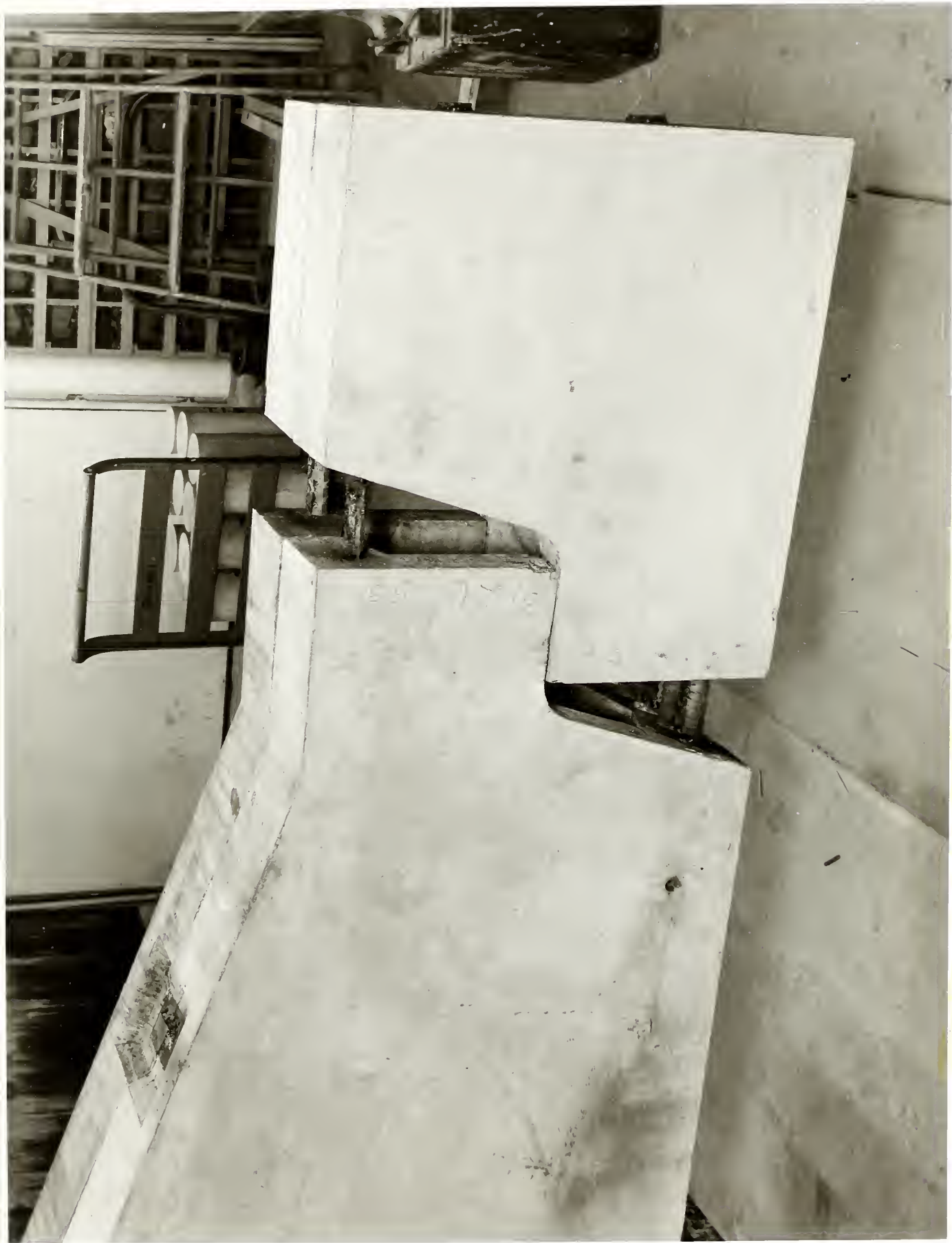
Fig. 2 - Close-up of girder splice.
