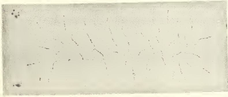
TYPE C ORDERED CRACKS (CRACKS SEEM TO FORM DEFINITE PATTERNS, RATHER THAN BEING RANDOM).
