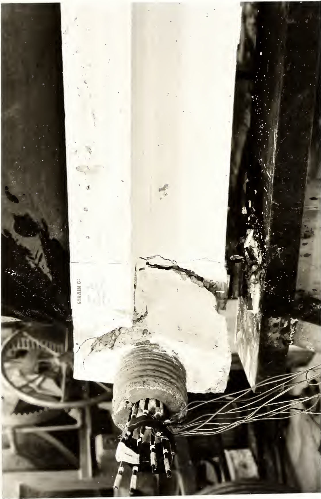
Fig. 12 - Close Up of Secondary Failure in N.E. Corner of Specimen.
