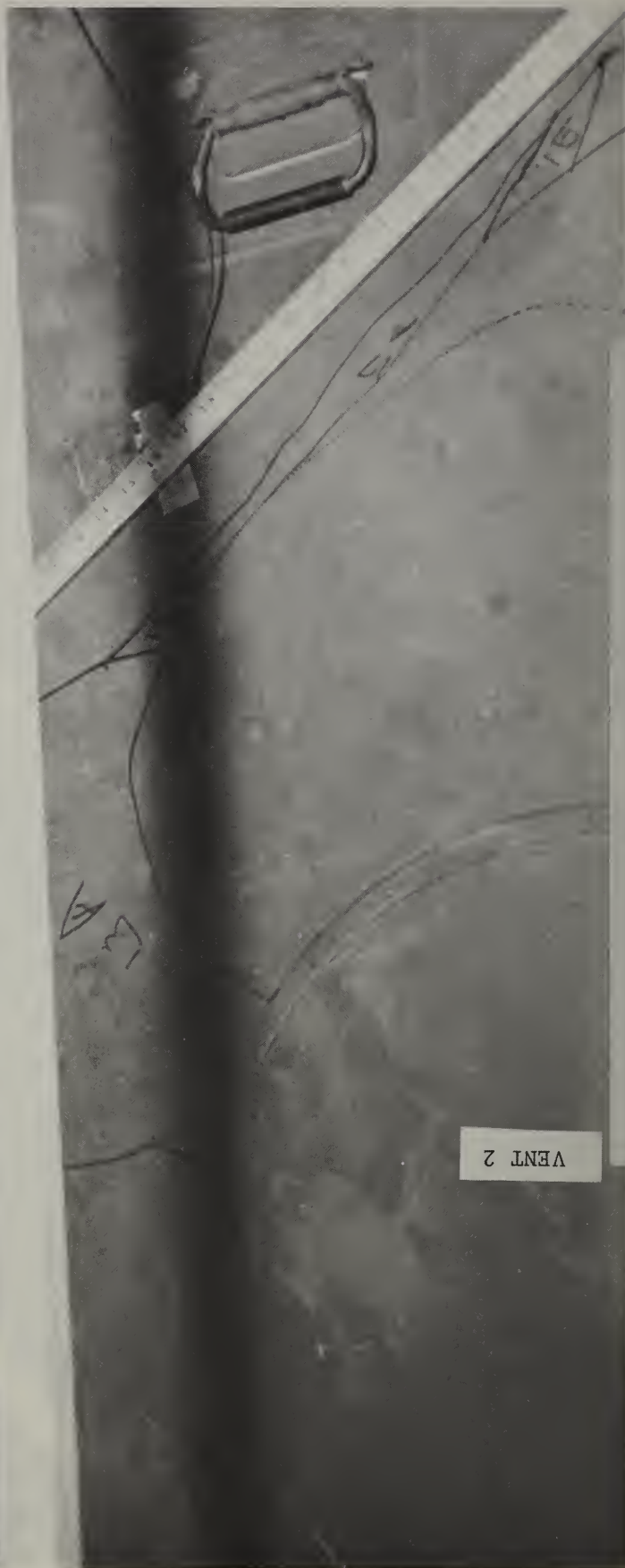
Figure 16. View of delaminated area around Vent 2, Ward B. See figure 13 for location.
