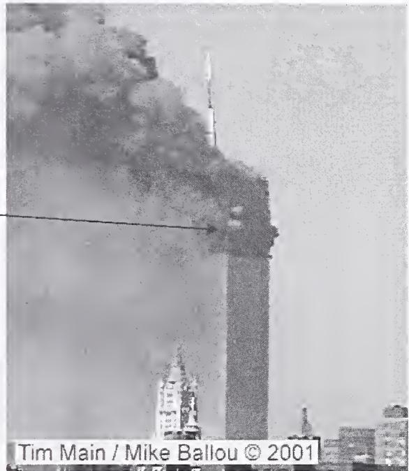
WTC 1 building section above impact damage zone tilts to the south
