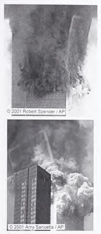
Figure 6–26. Kink on southeast corner near Floor 106 formed after collapse initiation.
