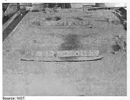
Figure 3–12. Sections cut through concrete slab to confirm extent and depth of spalling.
