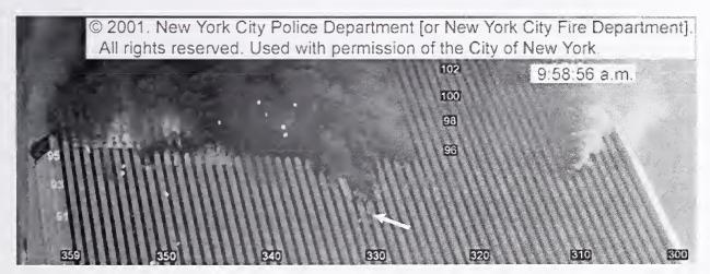
Figure 6–4. South face of WTC 1 with fire visible only on the west side at 9:25. Arrow shows region where debris pile under missing panel was observed.
