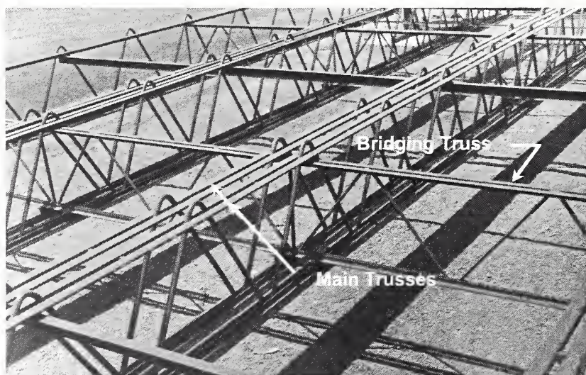
Figure 3–1. Mock up of floor truss system.
