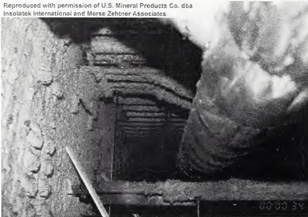
Figure 3-7. Connection of main truss to spandrel beam showing relatively thin SFRM on truss seat and no SFRM on damper.
