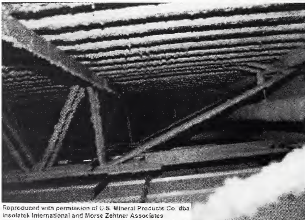
Figure 3-8. End of main truss showing low thickness of SFRM on truss members and no SFRM on damper saddle.
