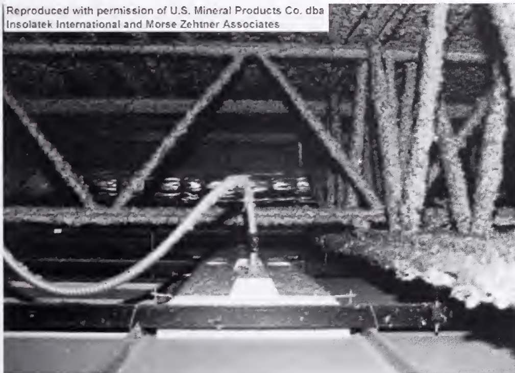
Figure 3–6. Intersection of main truss and bridging truss showing thinner SFRM on members of bridging truss.
