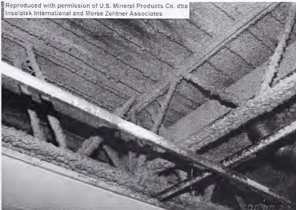
Figure 3–5. Intersection of main truss and bridging truss showing general good coverage of SFRM on truss members but thickness varies on web bars.
