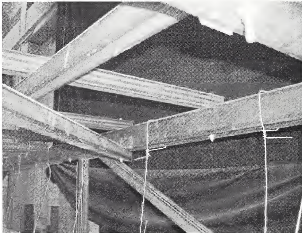
Figure 2–10. Connection of the roof to the main beams on the west side of the frame.
