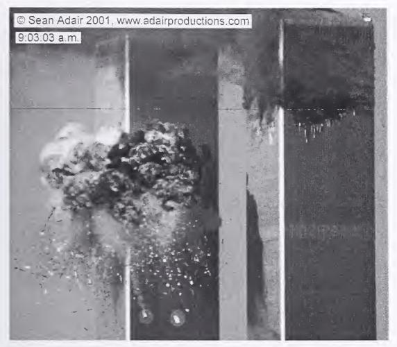
Figure 7-5. An image of the towers recorded from the north northeast is shown. The photograph was taken 4.3 s after the aircraft impact on WTC 2. Highlighted areas show two large pieces of aircraft debris that passed through the building and landed in the vicinity of the Church and Murray Streets intersection.
