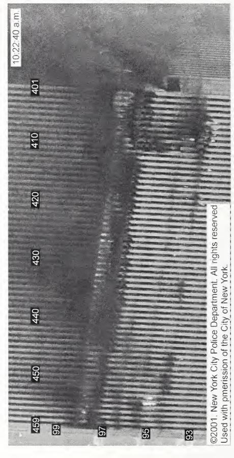
Figure 8-112. This cropped photograph was shot from a helicopter at 10:22:40 a.m. and shows the west face of WTC 1 from above. The image has been enhanced by adjusting the intensity levels, and column and floor numbers have been added.
