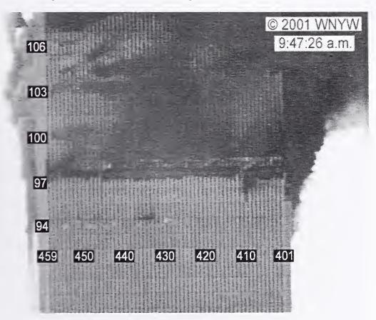
Figure 8-71. This image of the west face of WTC 1 is a frame captured from a video recorded by a news helicopter at 9:47:26 a.m. The image has been enhanced by adjusting the intensity range, and areas to the left and right of the tower are saturated.
