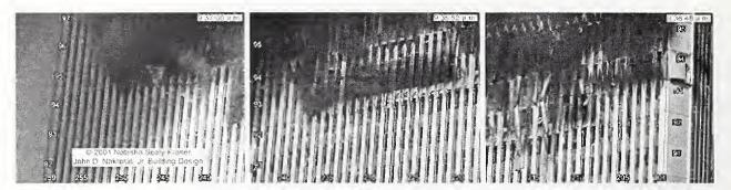
Figure 8-56. This series of three photographs shows various locations along the east face of WTC 1 around 9:37 a.m. Column and floor numbers have been added.
