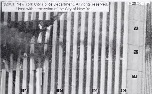
Figure 8-18. Two close-ups of the north face of WTC 1 taken from the photograph in Figure 8-17 show the east and west sides of the face around the 97th floor. The photos have been rotated, enhanced, and column and floor number have been added.
