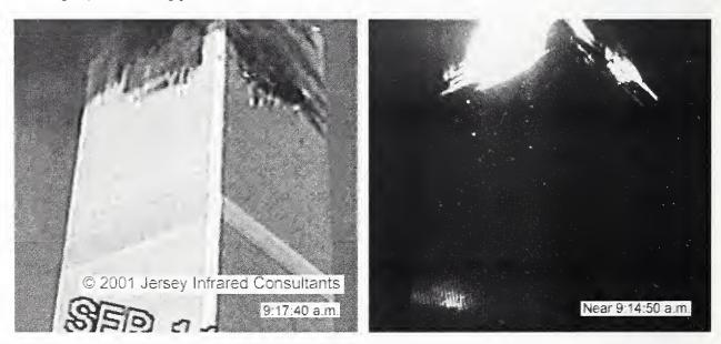
Figure 8-23. A frame from a standard video camera (left) and an image from an infrared camera (right) showing the north and east faces of WTC 1 are compared. The video frame was shot at 9:17:40 a.m., and the infrared image was taken around 9:14:50 a.m. (an uncertainty of 15 s has been assigned). The infrared image intensity levels were adjusted. The video frame has been rotated and sized to match the infrared image.
