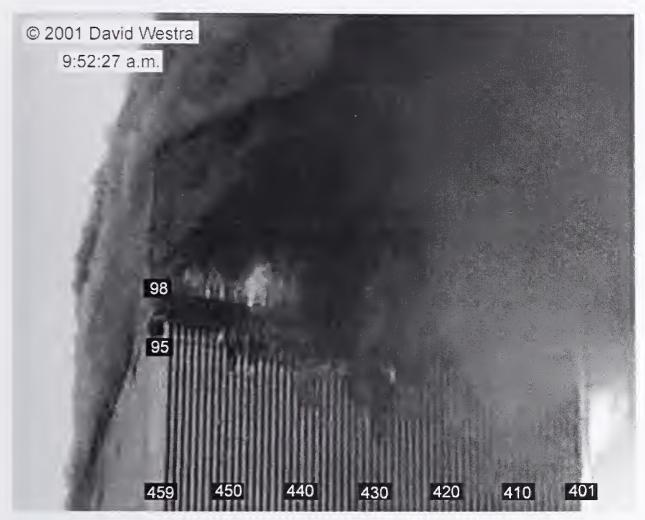
Figure 8-64. This cropped photograph shows the south face of WTC 1 at 9:52:27 a.m. The intensity levels have been adjusted and column and floor numbers have been added. For reference purposes, the missing aluminum panel on the southwest corner of the towers is on the 96th floor, and the heaviest fire is on the 98th floor.
