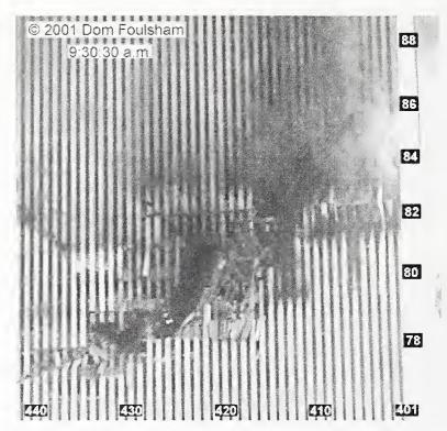
Figure 7-22. This cropped photograph shows the damage to the south face of WTC 2 caused by the aircraft impact. The image was enhanced by adjusting the intensity levels.
