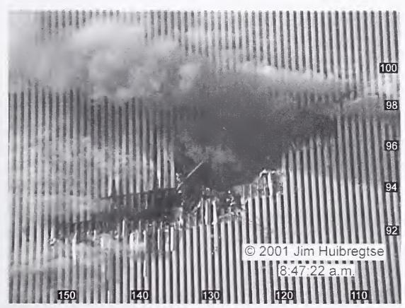
Figure 6-4. This image of the north face of WTC 2 is a frame taken from a video recorded at 8:47:22 a.m. Column and floor numbers have been added.
