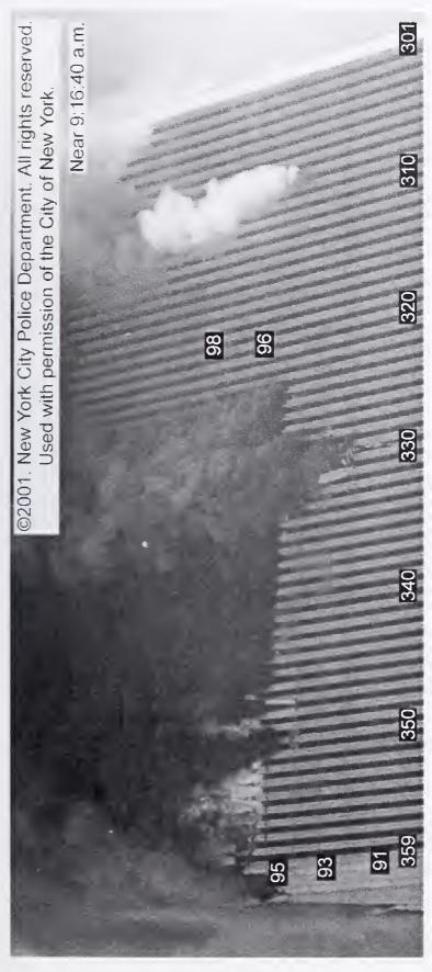
Figure 8-27. This image of the south face has been cropped from a high-resolution photograph. There is a 35 s uncertainty in the assigned time of 9:16:40 a.m. The image has been enhanced and rotated. Column and floor numbers have been added.
