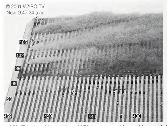
Figure 8-72. This view of the west face of WTC 1 was captured from a video recorded at 9:47:34 a.m. There is a 30 s uncertainty in the assigned time. The image has been enhanced by adjusting the intensity levels, and some locations above the building are saturated. Column and floors numbers have been added.
