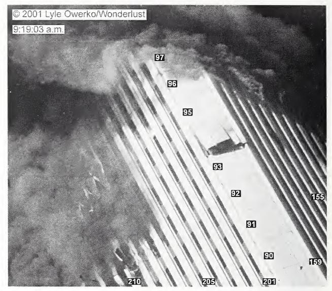
Figure 8-39. This cropped close-up photograph showing the northeast corner of WTC 1 was taken at 9:19:03 a.m. It has been enhanced, and column and floor numbers have been added.
