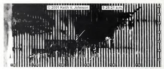
Figure 8-37. This cropped photograph shows the north face of WTC 1 at 9:28:21 a.m. The image has been rotated and enhanced. Column and floor numbers have been added.
