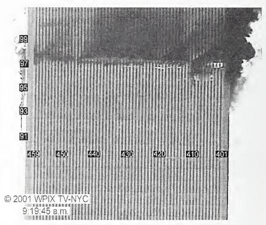
Figure 8-47. This image of the west face of WTC 1 is a frame captured from a video recorded by a news helicopter at 9:19:45 a.m. The image has been enhanced by adjusting the intensity range, and areas to the left and right of the tower are saturated. Column and floor numbers have been added.
