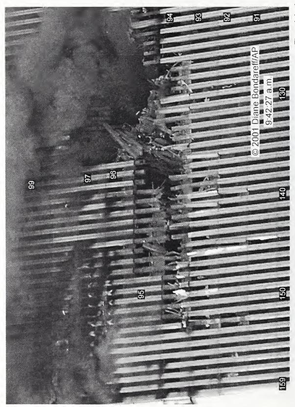
Figure 8-53. This sharp photograph shows the eastern portion of the north face of WTC 1 at 9:42:27 a.m. The original version has been cropped and enhanced. Column and floor numbers have been added.
