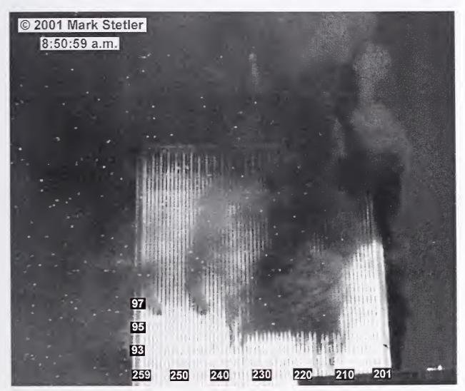
Figure 6-10. Photograph showing the east face of WTC 1 recorded at 8:50:59 a.m. Column and floor numbers have been added.
