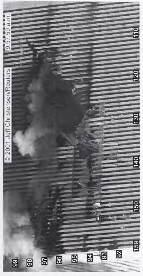
Figure 8-55. This image shows the north face of WTC 1 at 9:57:59 a.m. The original has been rotated, cropped, and enhanced. Column and floor numbers have been added.
