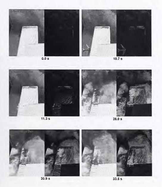
Figure 7-14. Frames from a composite video are shown. The half frames on the left are taken from a video showing the aircraft impact on WTC 2, while the half frames on the right are generated by subtracting a frame recorded prior to the aircraft impact from all subsequent frames in the original video. Times refer to the period since the start of the difference video.
