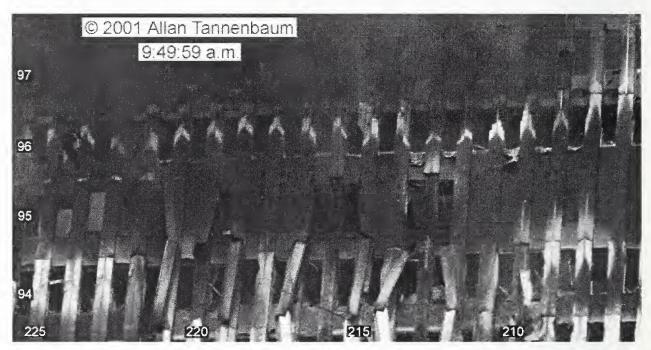
Figure 5-10. This cropped photograph shows a portion of the east face of WTC 1 at 9:49:59 a.m. The image has been rotated and enhanced by adjusting the intensity levels. A number of carets are visible near the tops of windows on the 96th floor. These carets were created during periods of external flaming from adjacent open windows. Column and floor numbers have been added.
