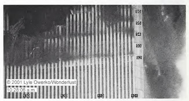
Figure 8-100. This cropped photograph shows a portion of the north face and an oblique view of the west face for WTC 1 at 10:28:06 a.m. The intensity levels of the image have been adjusted, and column and floor number have been added.
