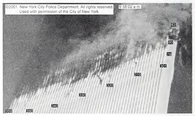
Figure E-16. This cropped image shows the east face of WTC 2 at 9:58:02 a.m. The intensity levels have been adjusted, and column and floor numbers have been added.
