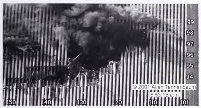
Figure 8-3. An enlargement of a portion of the photograph reproduced in Figure 8-2 showing the north face of WTC 1 at 8:53:15 a.m. is shown. Labels showing floor and column numbers have been added.
