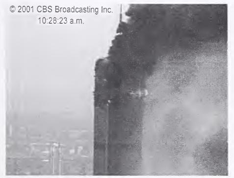
Figure 8-110. This image showing the south face of WTC 1 was taken from a video shot from a news helicopter at 10:28:23 a.m. The intensity levels of the image have been adjusted. Two areas showing flames that were pushed out of the tower as it started to collapse are highlighted.
