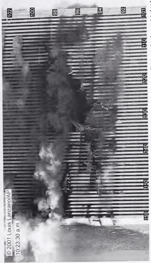
Figure 8-99. This cropped photograph shows the north face of WTC 1 at 10:23:30 a.m. The image has been rotated and enhanced by adjusting the intensity range. Column and floor numbers have been added.
