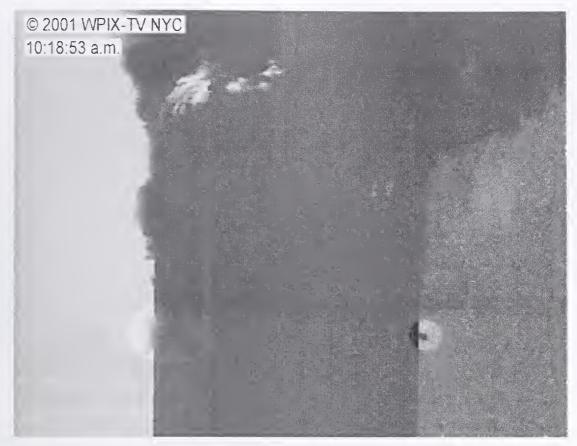
Figure 8-97. This image showing the west face and an oblique view of the north face was captured from a video shot from a news helicopter at 10:18:53 a.m. The highlighted areas with adjusted intensities indicate smoke and br dust plumes that were pushed from the north and south faces by a pressure pulse that passed through the tower at 10:18:48 a.m.
