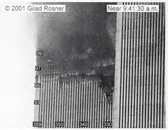
Figure 8-61. This untimed photograph shows the south face of WTC 1. It is estimated that it was taken between 9:40:40 a.m. and 9:42 a.m. Column and floor numbers have been added.
