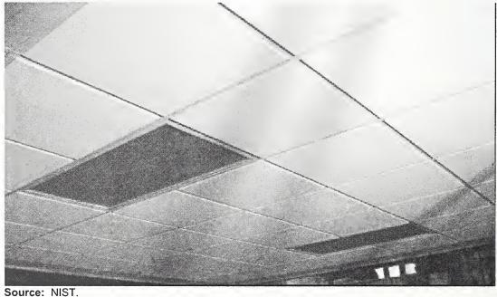
Figure 3–1. Top and bottom views of a ceiling system similar to that originally installed in the tenant spaces.
