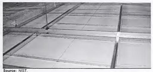
Figure 3–2. Bottom and top views of a ceiling system similar to that originally installed in the core areas.
