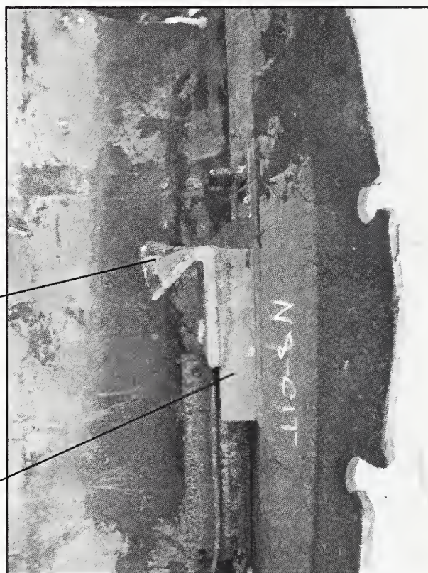
Figure A1b: Type A floor truss connector
