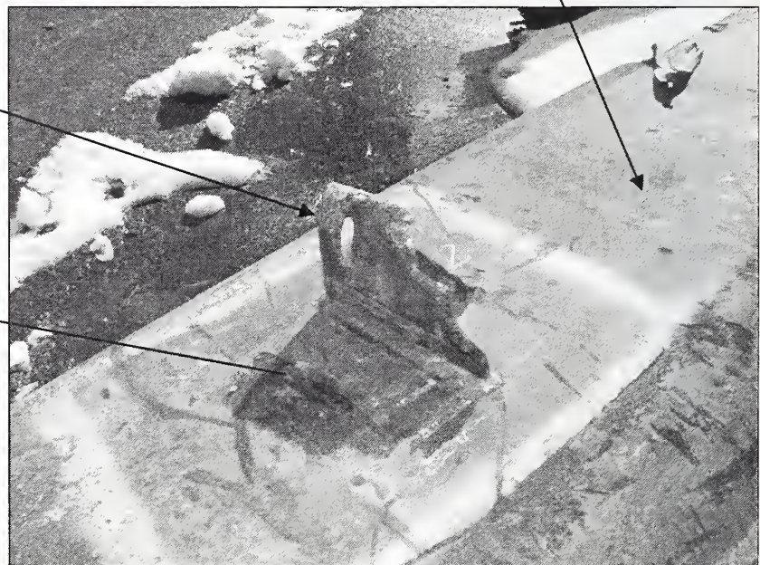
Figure A2b: Type B floor truss connector
