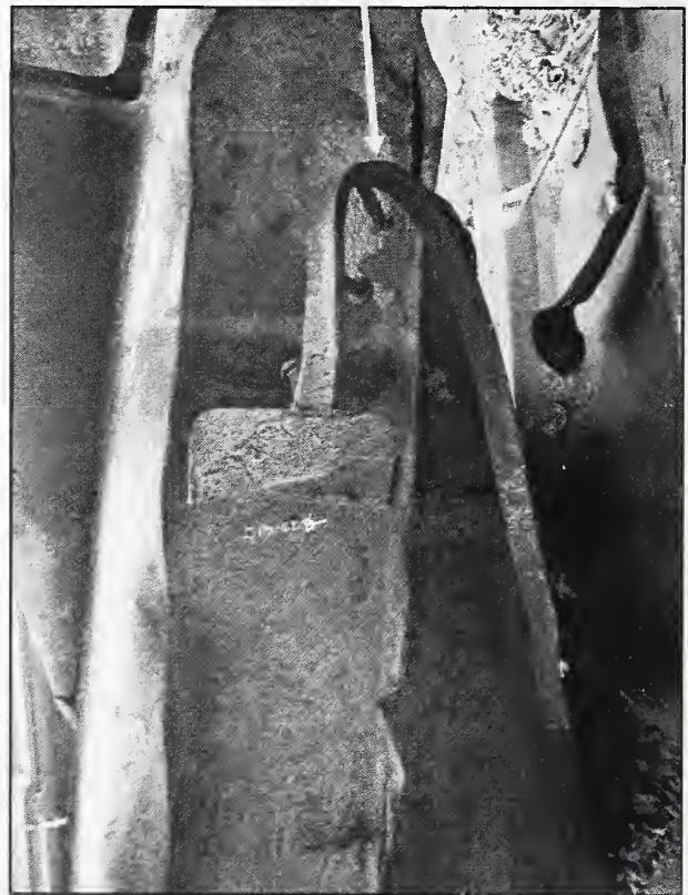
Figure A3d: Type C floor truss connector
