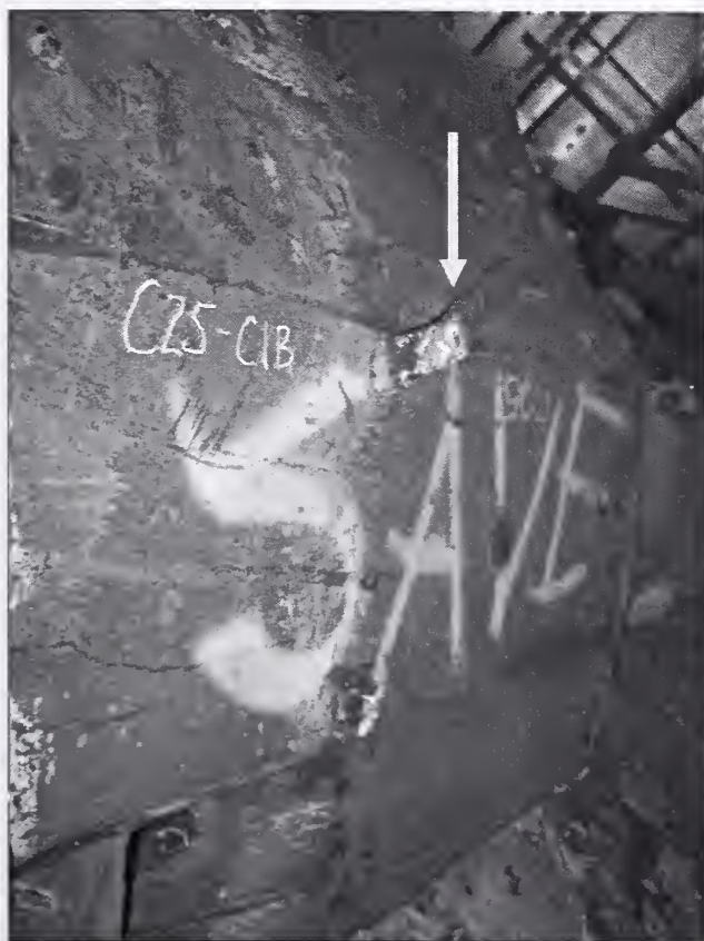
Figure A4a: Type D floor truss connector
