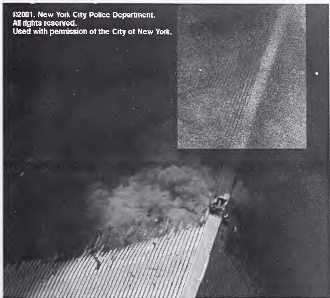
Figure 2-46. Image of the NE corner of WTC 2, several seconds before collapse. The corner shows no distortion of the type in the previous figure. This would imply that the distortion accompanied the collapse and did not precede it. The region in the upper right is enhanced for visibility.
