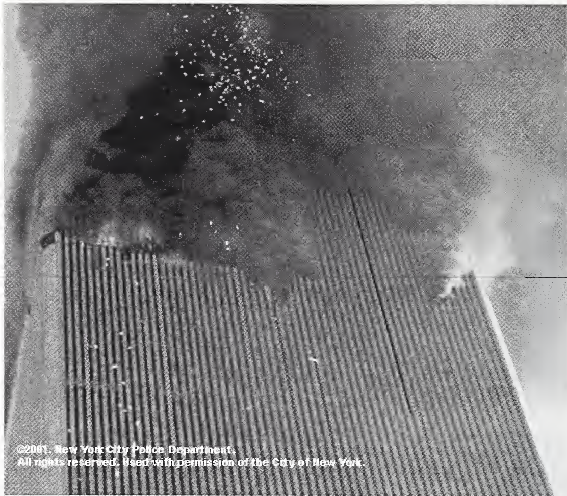
Figure 2–26. South face of WTC 1 58 min after (9:25 a.m.), showing no bowing in the outer columns.
