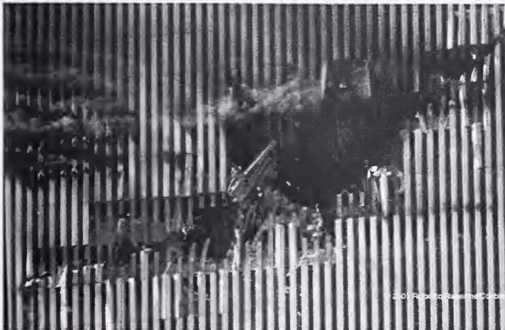
Figure 2–7. Unenhanced image Corbis_NRM161282 showing the impact hole in the north face of WTC 1.
