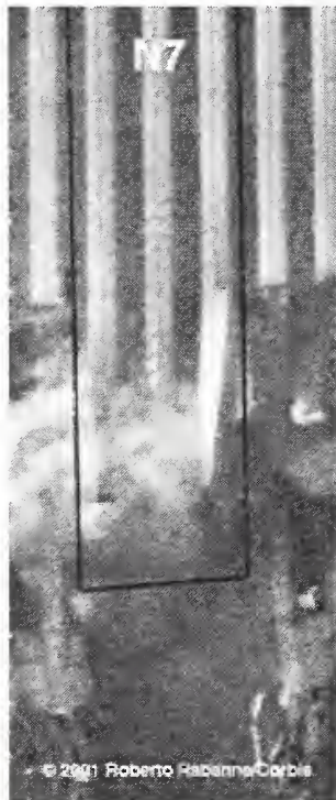
Figure 2-18. Close-up of pre-collapse condition of panel N-7 (A127: 97-100).
