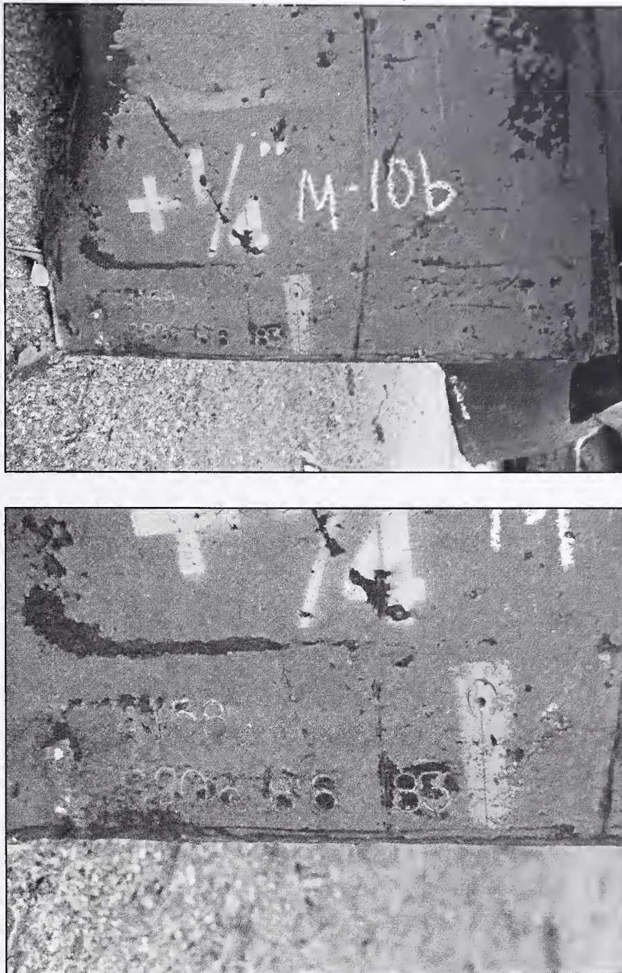
Figure 3–3. Example of stampings on the interior base of the middle column for each panel.
