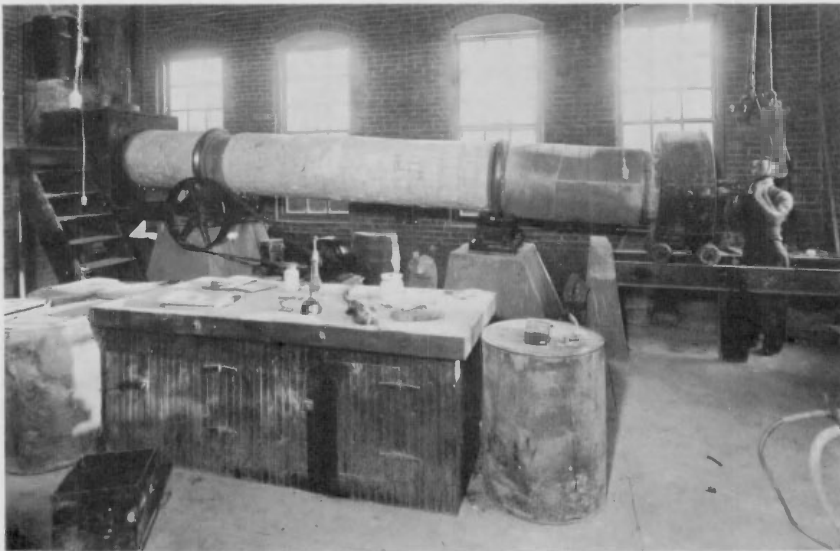
Above, the NBS small-scale experimental paper mill in which all the operations of paper-making could be studied under controlled conditions. Below, the rotary cement kiln at the Pittsburgh laboratory, brought to Washington in 1918, for determining the effects of various processes in the manufacture of cements.
