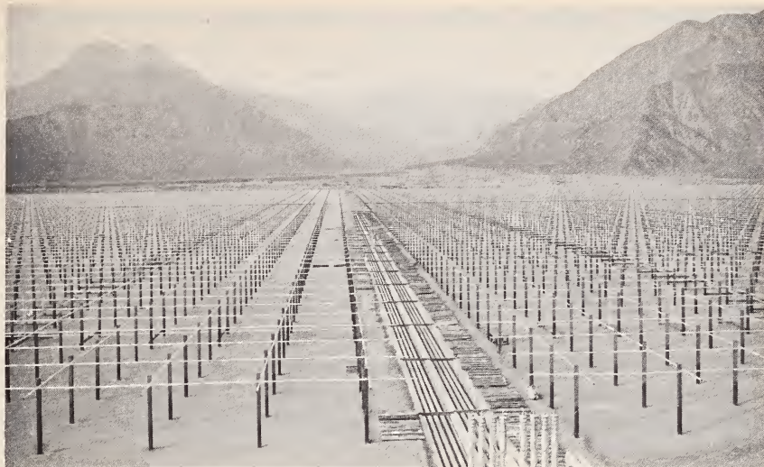
The 22-acre antenna of the Jicamarca Radar Observatory near Lima, Peru. This radar, in full operation since December 1962, has recently been re-instrumented to measure electron density profiles using the Faraday effect. These instruments also provided information on electron and ion composition and temperatures from 200 to 1200 km. (See page 219)
