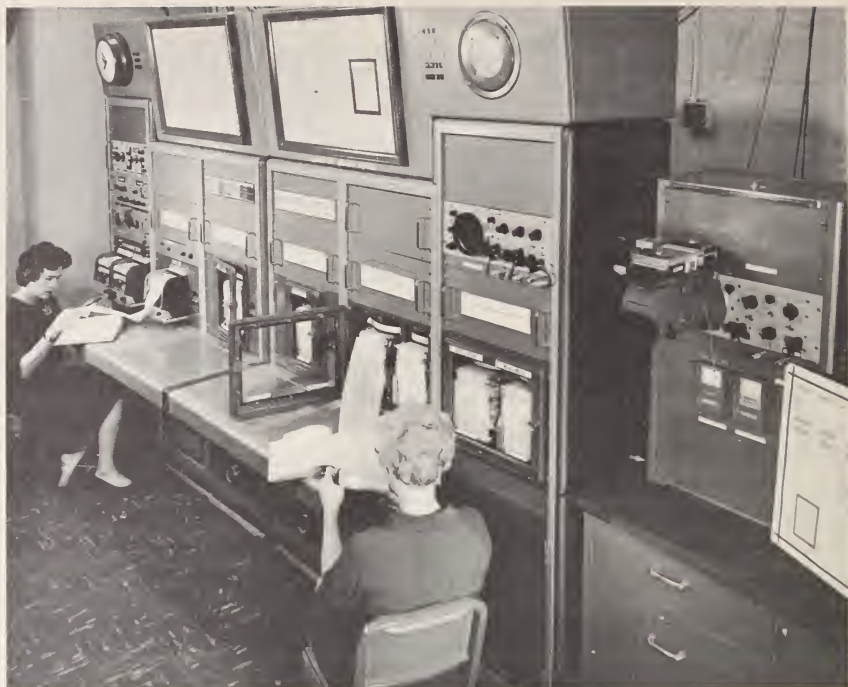
Equipment used for the international comparison of atomic frequency standards using the VLF signals of Radio Stations GBR (England) and NBA (Canal Zone). Such studies showed that atomic "clocks" in England, France, Switzerland, and Canada agreed with those at NBS Boulder to within 3 parts in 10^{10} . (See page 109)
