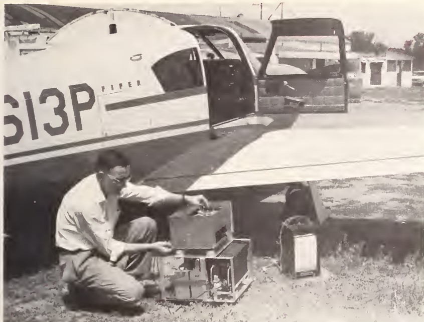
Airborne refractometer equipment used in studying the effects of atmospheric inhomogeneities and turbulence on missile radioguidance systems using microwaves (page 130).
