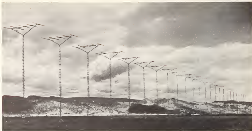
Array of 25 Yagi antennas used to pinpoint the direction of radio signals received from "forward scatter" transmission (page 136).
