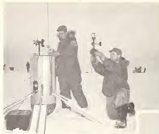
Right: The anchored, unmanned, automatic weather station, "Nomad," developed for the Navy, was the first automatic weather station to detect formation of a hurricane. Above: NBS engineers also helped the Navy to develop and set up a chain of automatic weather stations in the Antarctic (page 120).
