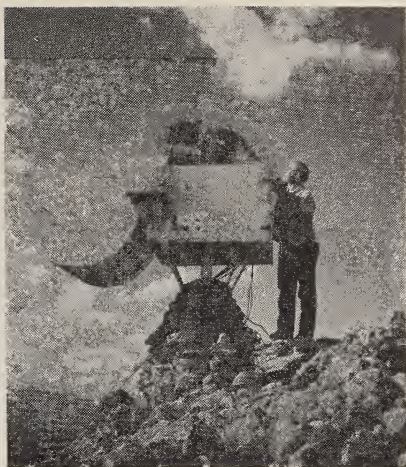
Automatic telescopic photometer installed on Fritz Peak in the Rocky Mountains for observation of night airglow (p. 91). A built-in programming unit causes the photometer to scan the night sky continuously. Six photometers have been designed and constructed for the International Geophysical Year.
