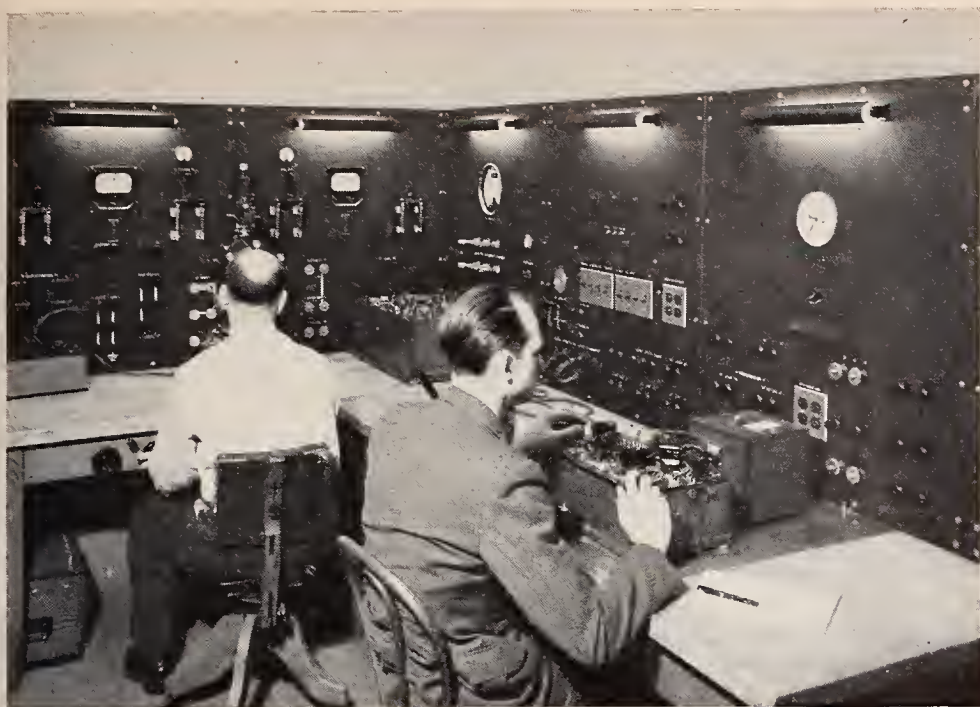
NBS laboratory in which ammeters, voltmeters, and other electrical indicating instruments are calibrated in terms of the national standards of resistance and voltage.
