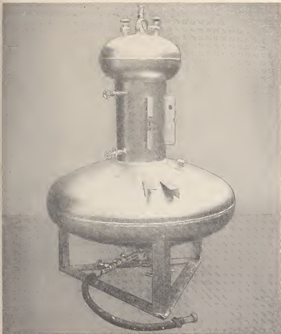
FIGURE 13. Volumetric-type LPG-meter prover—State of Florida.
