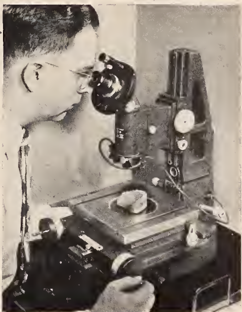
Laboratory studies of the fundamental physical and clinical properties of dental materials are conducted at the Bureau (p. 13). Top: tendencies toward shrinkage in dental amalgam are determined by means of the dental interferometer. Lower left: to obtain data on materials and techniques, experimental dentures are processed under controlled conditions. Lower right: measurement of shrinkage in a plastic denture.
