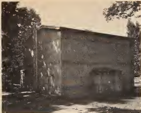
Left: test bungalow constructed at the Bureau for research in heat transfer phenomena in small houses. This bungalow has since been completely enclosed within an insulated enclosure (right) so that the temperature outside of the house can be maintained at any temperature condition encountered throughout the United States.
