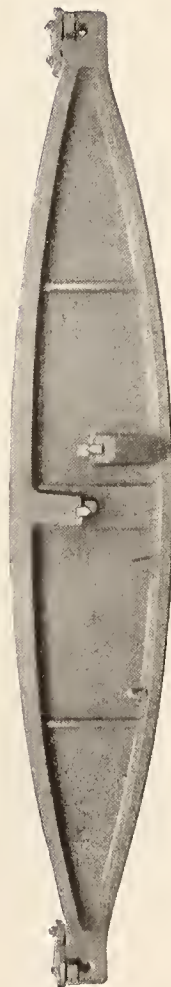
FIG. 8.—Middle extension lever.
