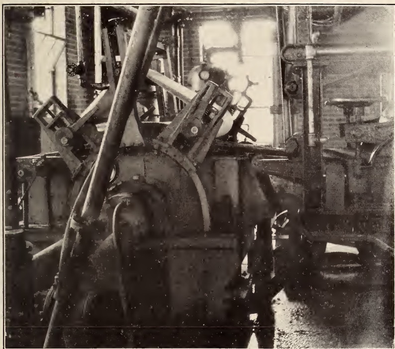
FIGURE 10.— Mat-forming machine
