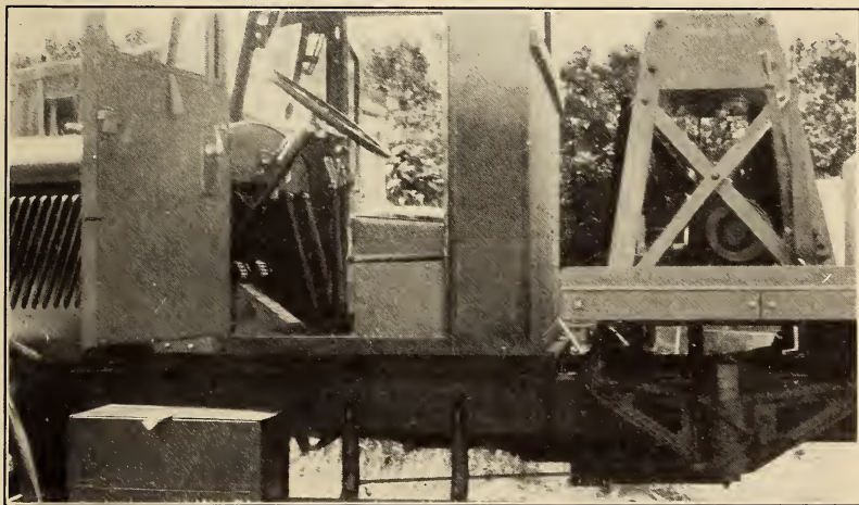
FIGURE 10.—Detailed view of cab and hoisting unit
