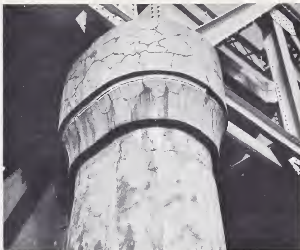
FIGURE 3. King City Bridge. Pier cap with typical map cracking.
