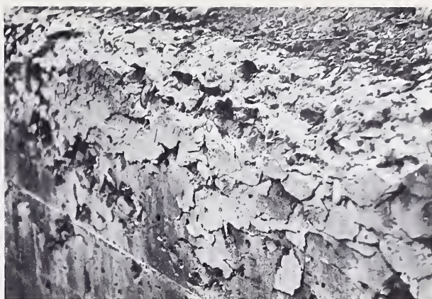
FIGURE 10. Frost damage to green concrete containing porous aggregate.
