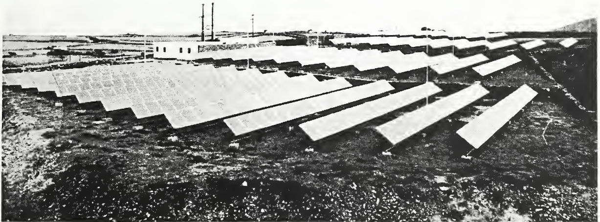
3-1 Overall view of the Kythnos photovoltaic plant
