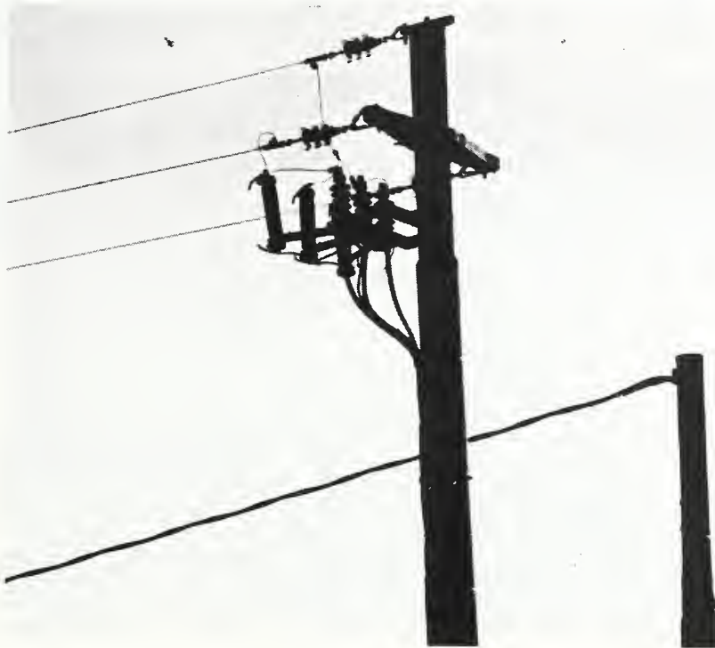
2-13 Surge arresters at 20 kV interface
