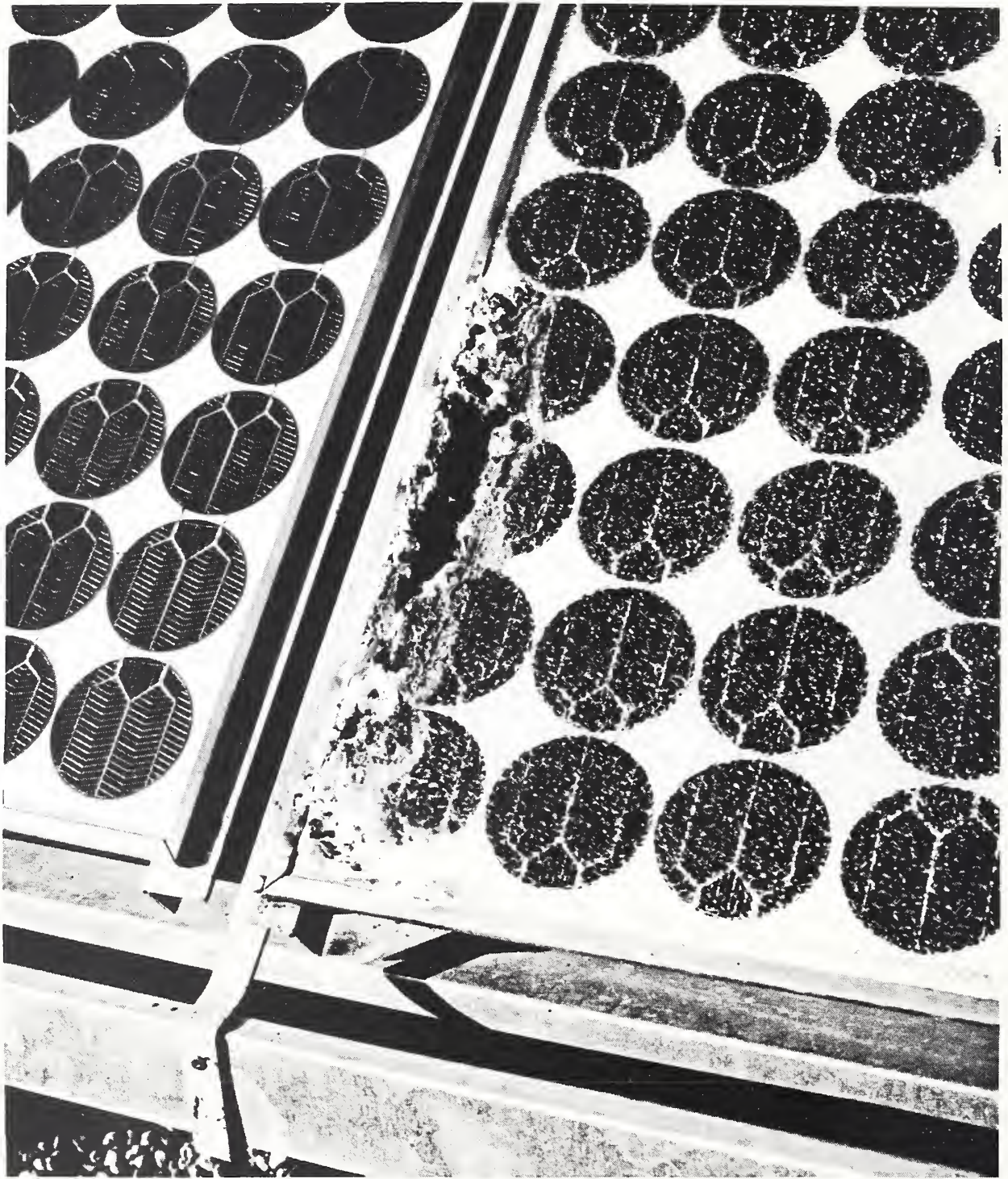
2-2 Damaged panel, attributed to lightning
