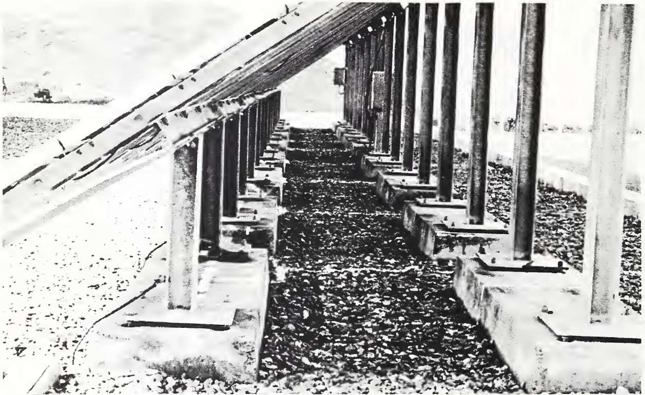
2-6 Side view of array and columns
