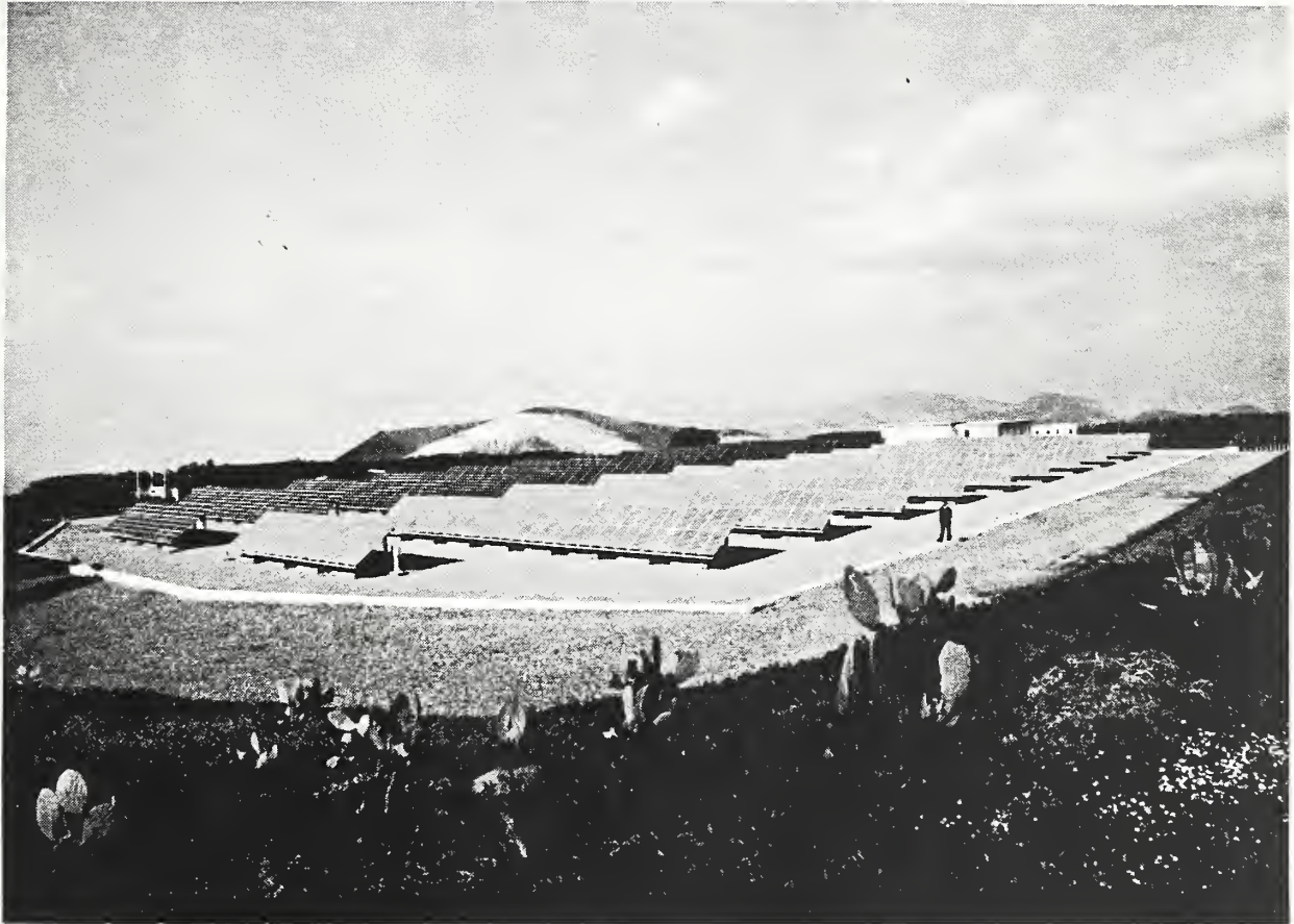
2-1 Overall view of the Vulcano photovoltaic plant
