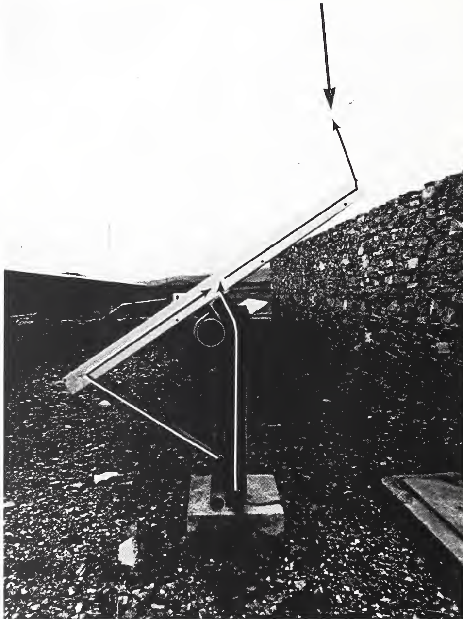
3-39 Side view of array, with hypothetical current paths to ground
