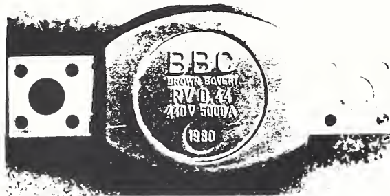
Figure 3: Surge arrester for 220/440 V circuits, service entrance installation
