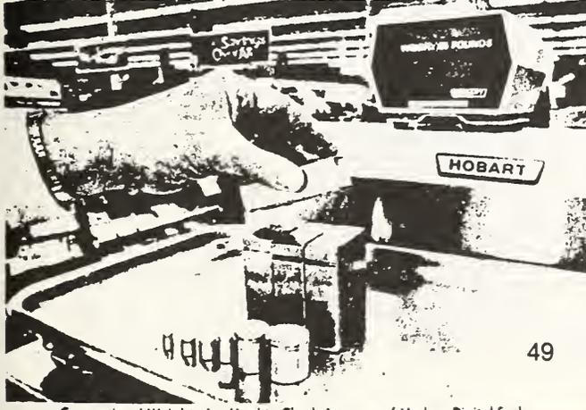
Conventional Weights Are Used to Check Accuracy of Modern Digital Scale
