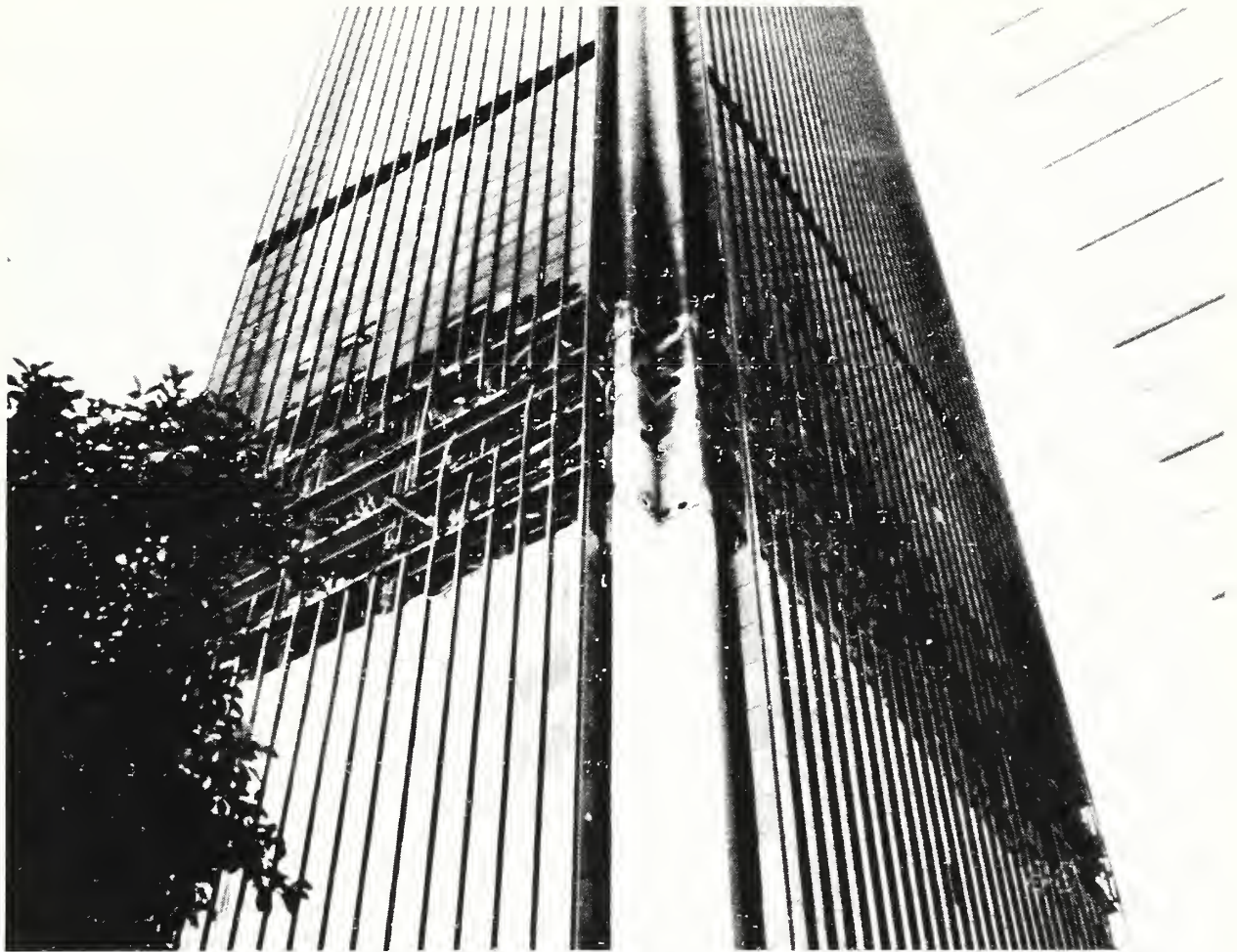
First Interstate Bank fire, Los Angeles, CA, May 4, 1988.
