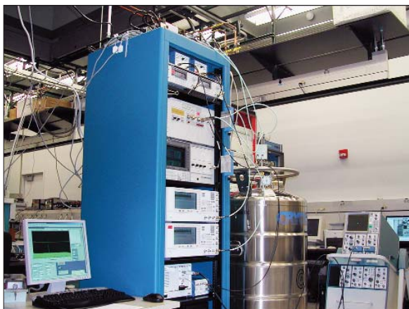
Figure 3. ACJVS system installed at NIST-Gaithersburg.
