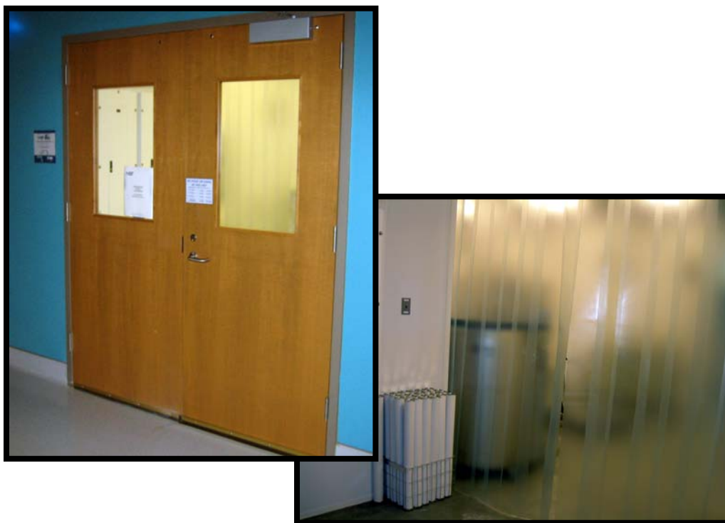
Figure 8. Double Doors and Vinyl Strip Shield Curtain in the ISO Class 7 Clean Room
