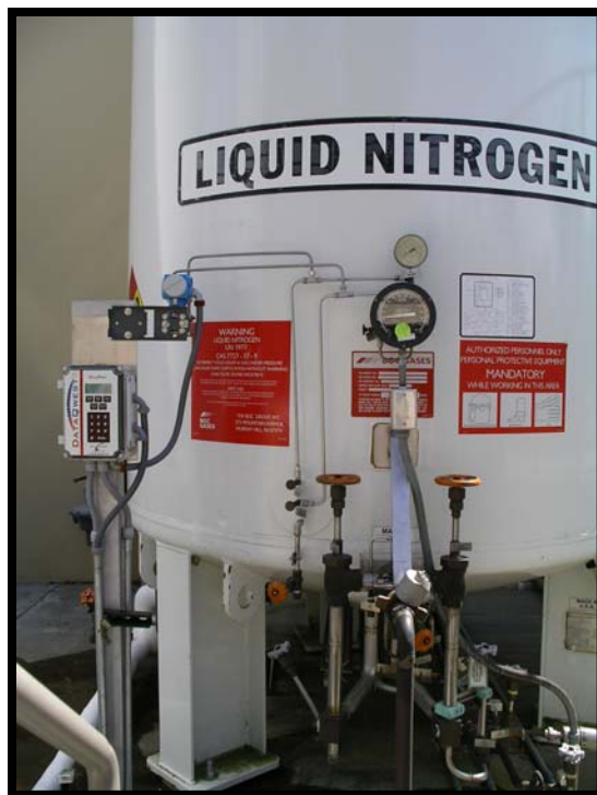
Figure 5. Marine ESB Vertical Liquid Nitrogen Storage Tank
