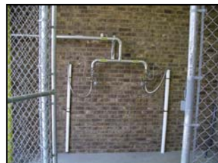
HML Liquid Nitrogen Fill Station
