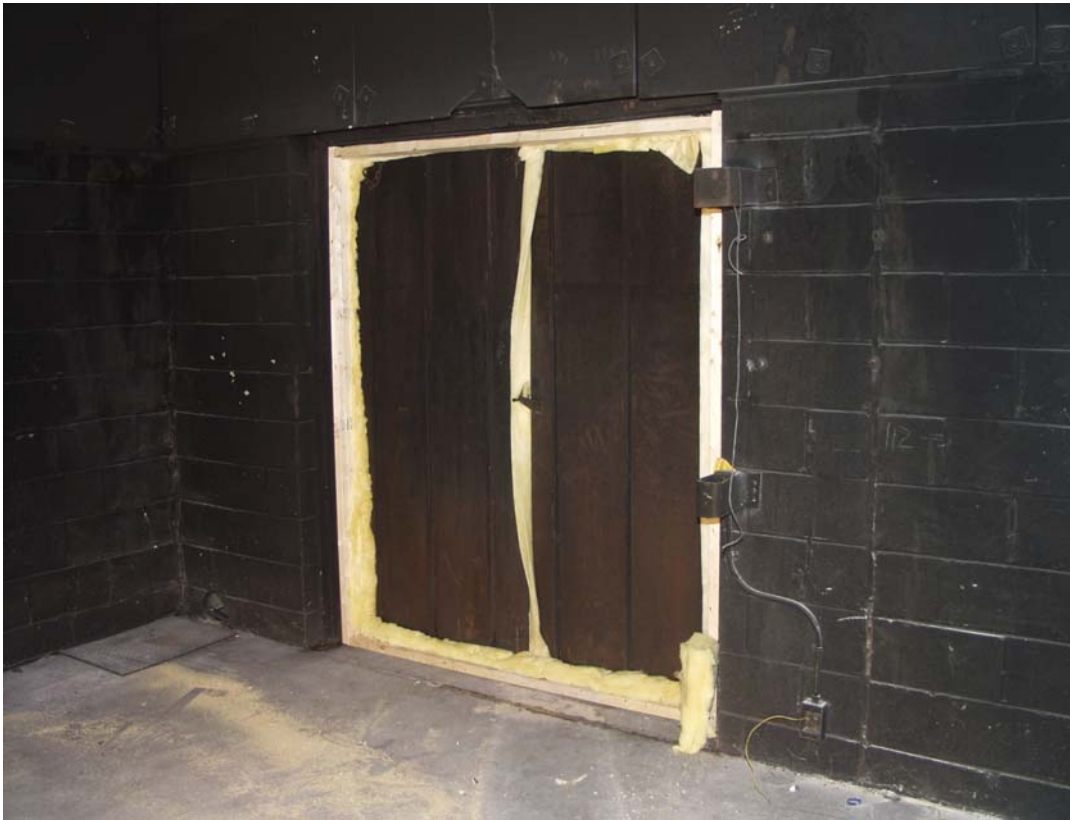
Figure 4. Door D3 Sealed with Wood Frame and Insulation
