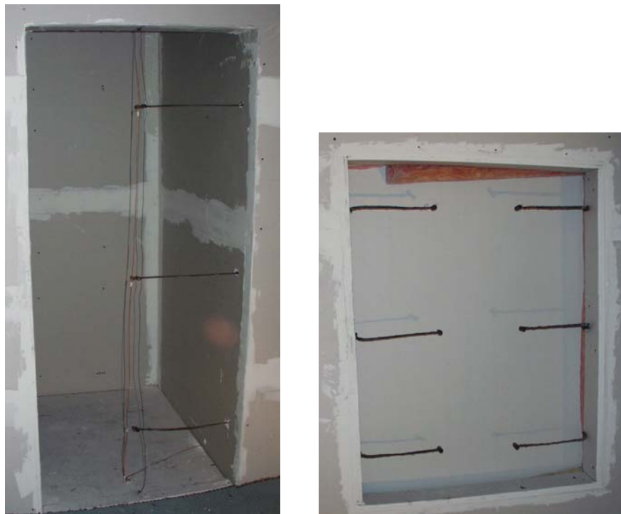
Figure 4-7. View of Doorway From Inside the Room into Corridor and Window with Instrumentation
