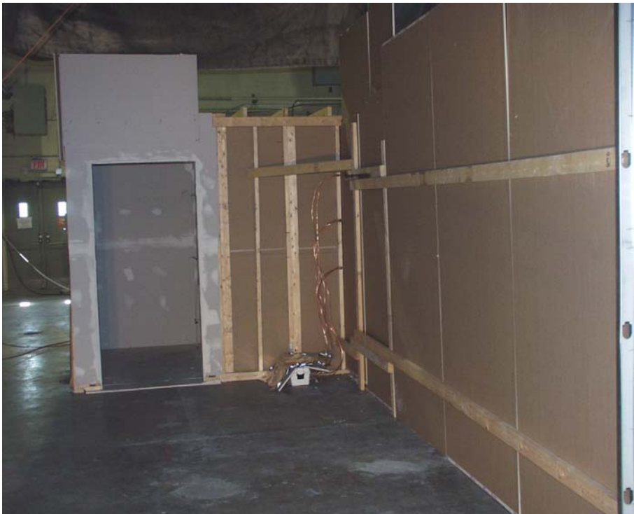
Figure 4-3. External View of Open Corridor Doorway
