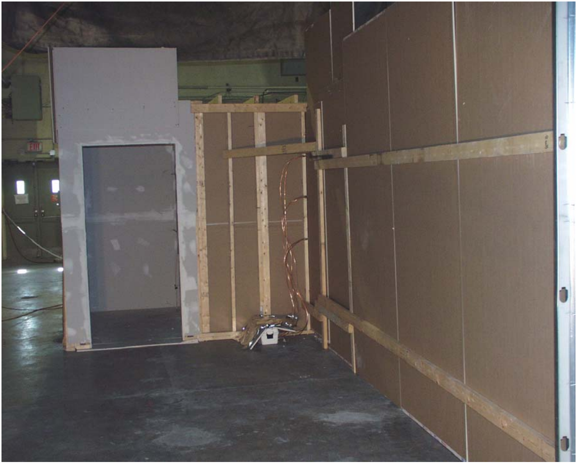
Figure 5 – External view of open corridor doorway
