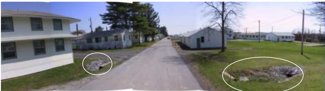
Figure 14 View of a culvert, the most frequent cause of emergency stops in the urban test area.
