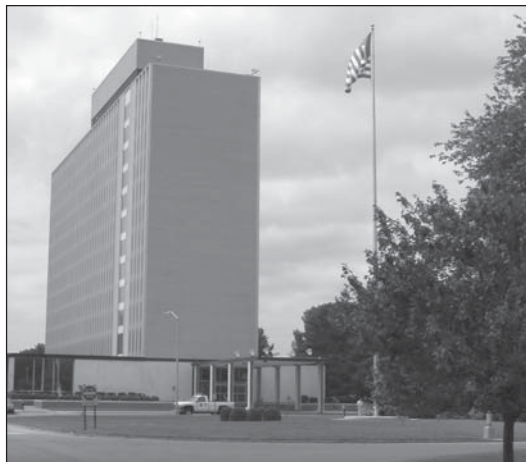
NIST’s 11-story Administration Building.
