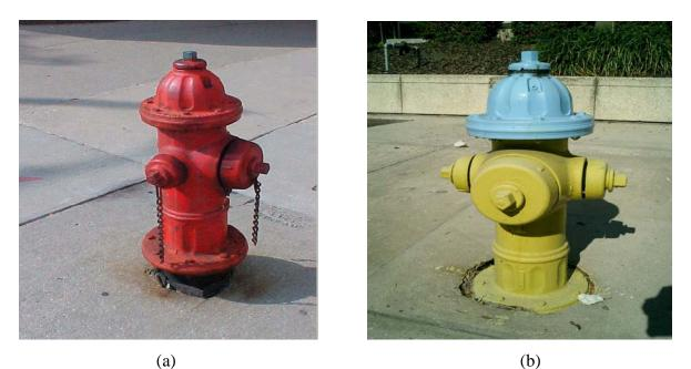
Fig. 2: Pictures of Standard Fire Hydrants (a) Side view of a three-nozzle hydrant showing the main nozzle or pumper connection  $(4^{1/2})$  diameter with 4 threads per inch), and one of the two small hose nozzles or hose connections  $(2^{1/2})$  diameter with 7<sup>1/2</sup> threads per inch), (b) Front view of a two-hose and one- pumper nozzles hydrant. (Reuter: Mike Hassler)
