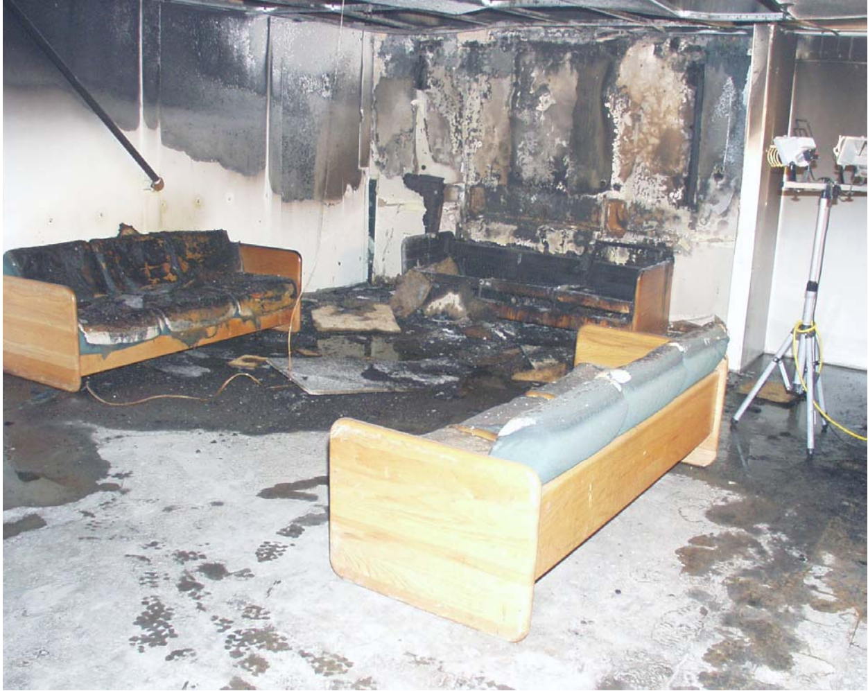
Figure 13. Photograph showing the day room after experiment 2.
