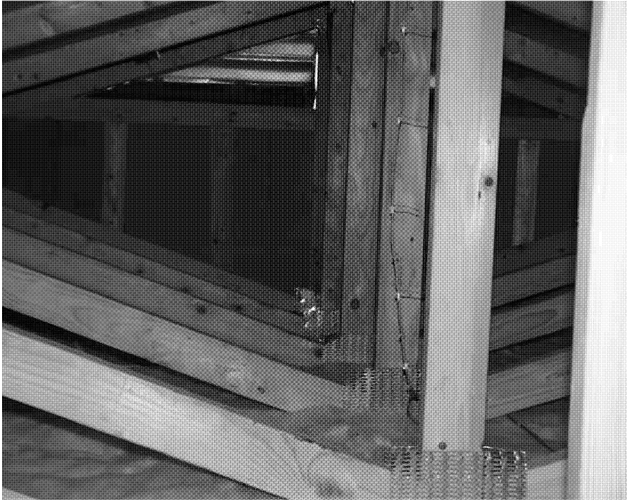
Figure 11. Photograph showing trusses supporting the roof structure with thermocouple array visible in front of second vertical wood member.
