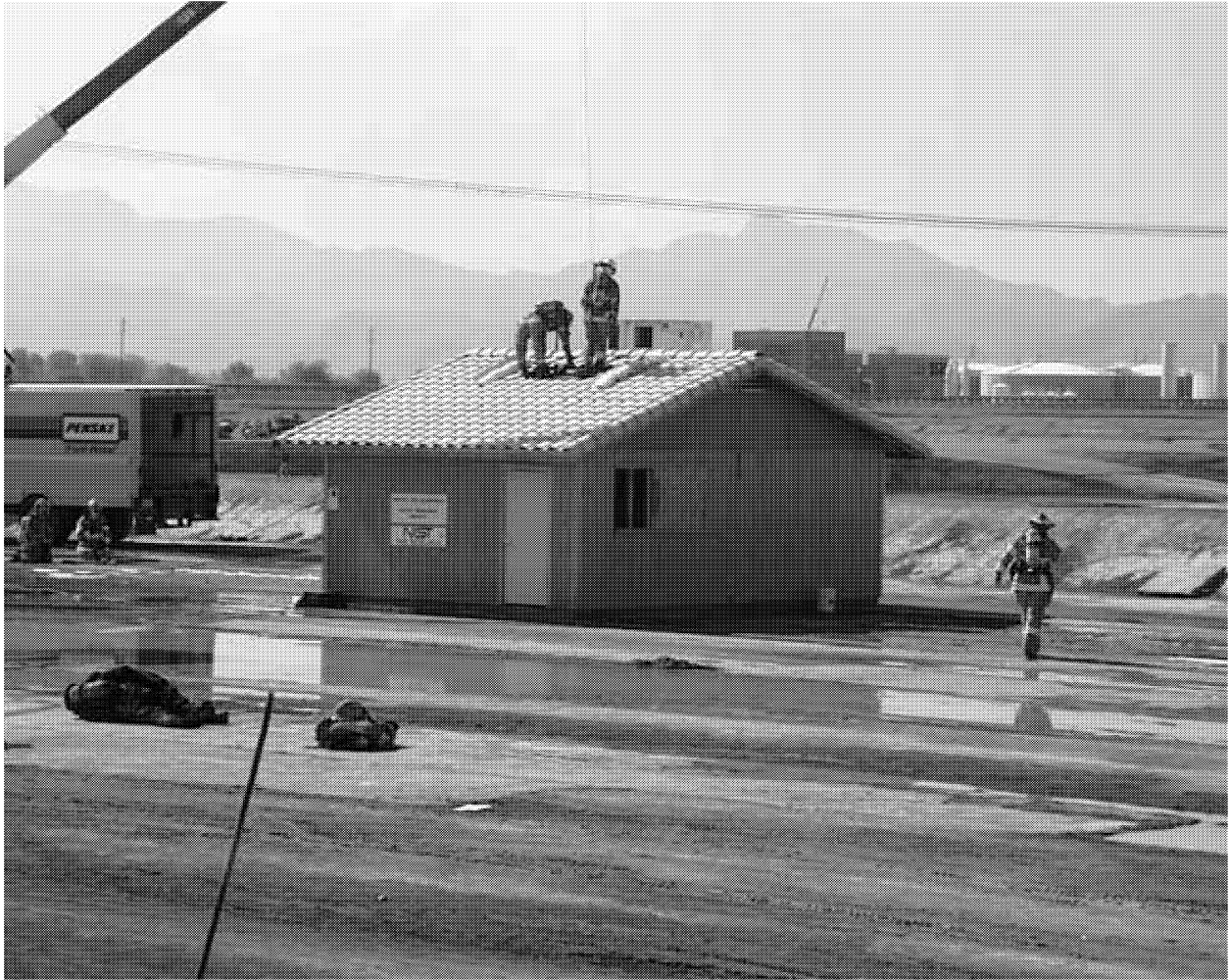
Figure 1. Photograph showing the front and one side of test structure with tile roof prior to start of test.
