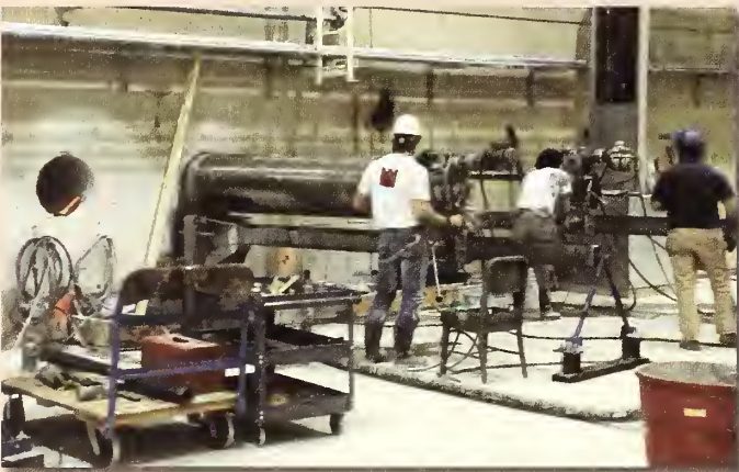
Drilling through 20' concrete wall to bring neutron guides from the source, 1989.
