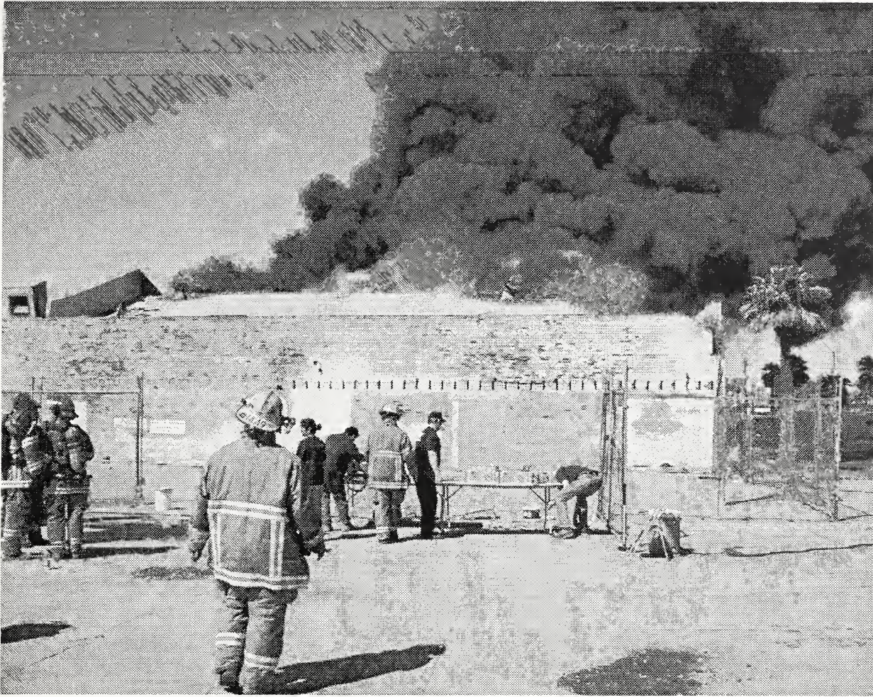
Figure 11. Photograph showing fire involving significant portion of roof structure with partial collapse beginning.
