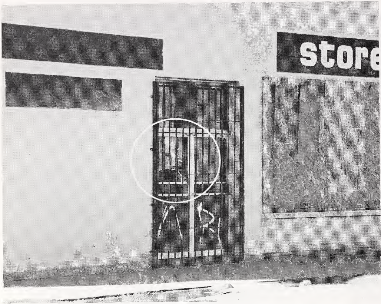
Figure 8. Photograph of front of warehouse with flames visible through front door at the start of the first test.
