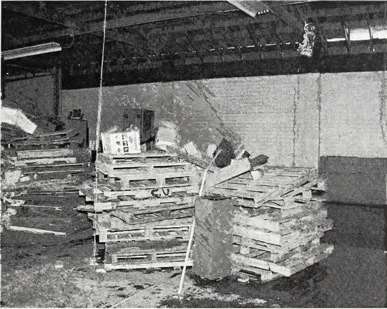
Figure 7. Photograph showing placement of wood pallets and adjacent thermocouple tree in the portion of the warehouse used for the second test.
